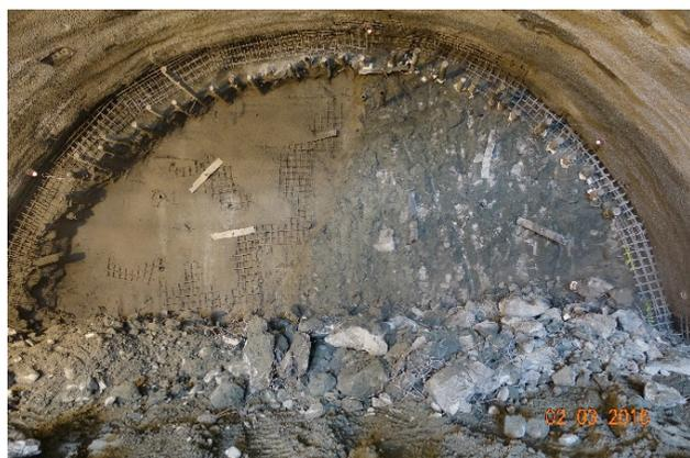
Figure 15: Grey moraine in the right side is excavated in one section. Brown moraine in upper left side is supported by sprayed concrete, wire mesh and face bolts.
