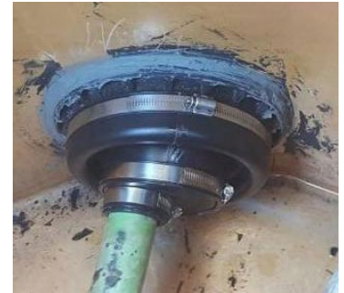
Example of Blueline Large KFD Repaired
