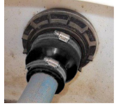
Example of OPW CS Medium Repaired
