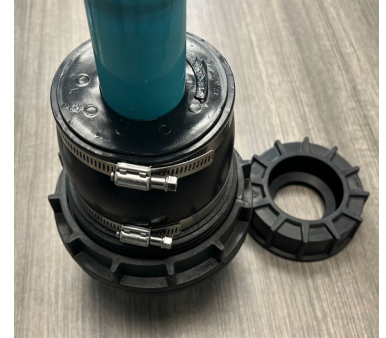
Example of APT Repaired
