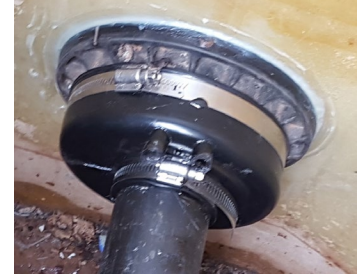
Example of Blueline Medium KFD Repaired
