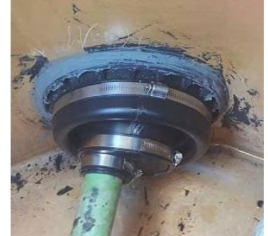
Example of Blueline Large KFD Repaired
