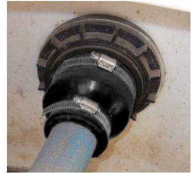
Example of OPW CS Medium Repaired
