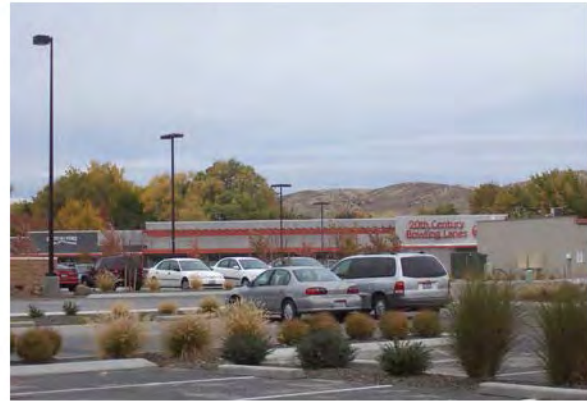
Façade and landscape enhancements were used to revamp this strip center on State Street.
