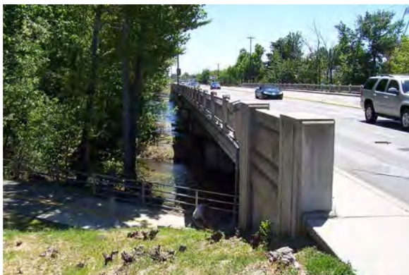
The 1956 Broadway Bridge
