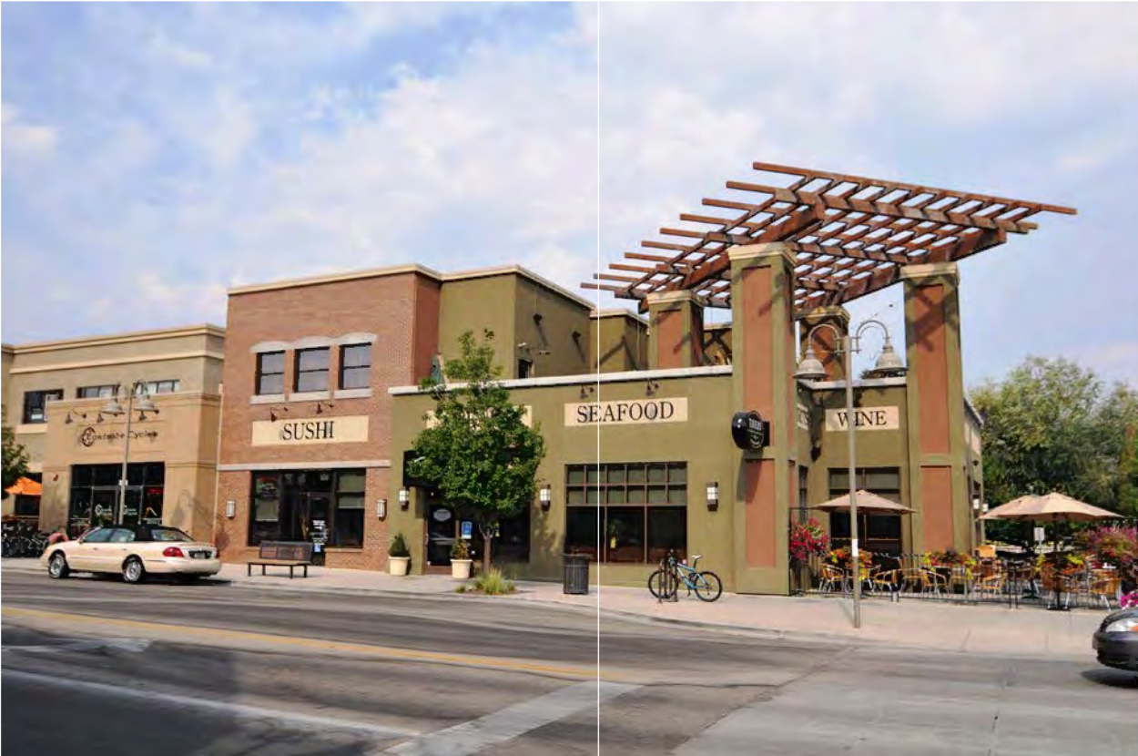
Bowen Crossing has grown and created an activity center that is a prime example of desirable mixed use design principles in this plan.
