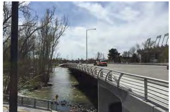
The 2016 Broadway Bridge
