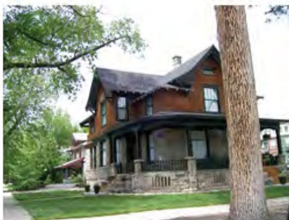
The city’s many historic buildings contribute to the image and identity of the community and its neighborhoods.
