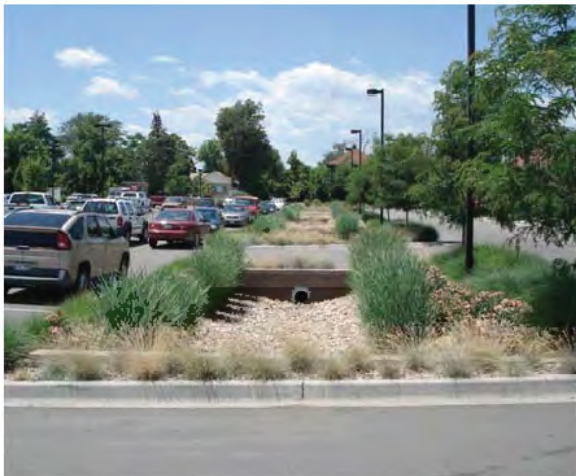
On-site stormwater improvements help reduce the amount of water in the city’s system during high precipitation while also removing pollutants.
