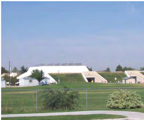
Amity Elementary School is designed with earth cover as well as solar panels.
