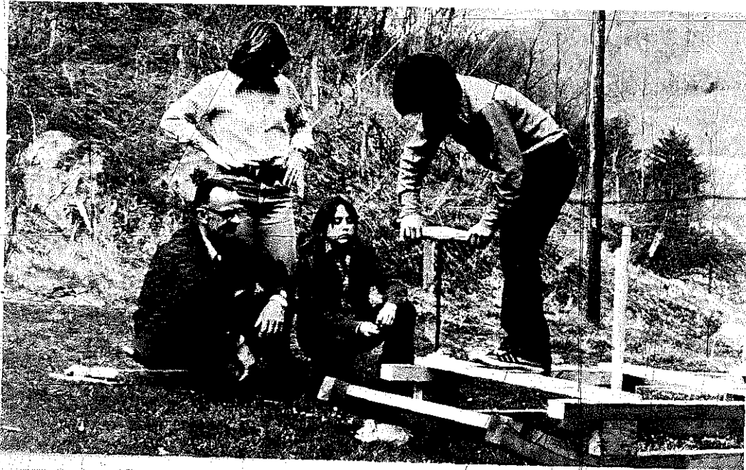
PLATE 172 With the 1" auger, Dwayne drills down through the oak crosspieces, the sills, blocks, and well into the runners. Long dowels driven into each of the six holes hold the sled together and keep such loads as logs from rolling off.
