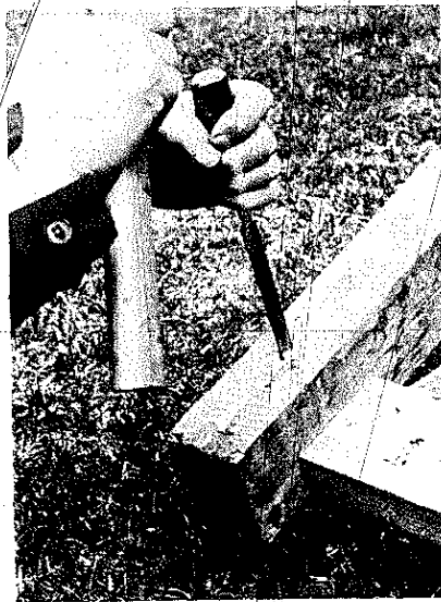
PLATE 169 After the bottoms of the pegs are sawed off flush, Tedra splits the bottom of each peg. Then he drives a wedge into the split to make the peg bind firmly in the hole.
