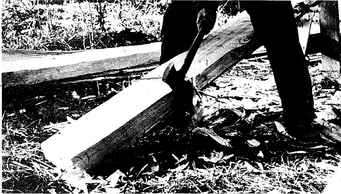
PLATE 409 From the center of the log, he measures off the width he wants the beam to be, flips two chalk lines as guides, raises the log onto sawhorses, and slices off the sides with an axe. He first scores the sides, then goes back and hews to the line.
