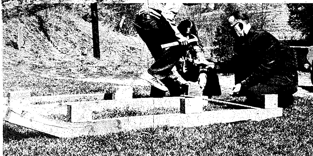
PLATE 166 The last block goes on. The wooden strip in front of Tedra's left hand has been nailed on temporarily to hold the runners the correct distance apart.
