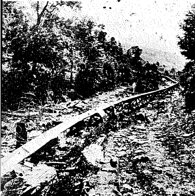
PLATE 271. Acid wood (chestnut) was essential for the production of paper. Companies like Champion International would build miles of flumes up into the mountains in order to get this acid wood out. A flume would begin high in a watershed nearly at the head of the creek. A splash dam at the head of the flume would hold water to be turned into the flume. The chestnut would be cut into five-foot lengths and split up and stacked beside the flume at intervals along its length during dry weather. Then, in wet weather when the stream was running full, water would be turned into the flume at the splash dam and the split wood would be loaded into it and carried to its end. The flume pictured here was on Big East Fork. (Photo courtesy of Champion Paper, a division of Champion International Corp., furnished by C. W. Hardin.)
