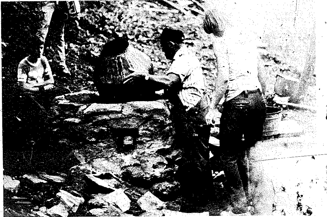
PLATE 436 When the rock sides were high enough to reach the cape of the still, Buick set it back into place.
