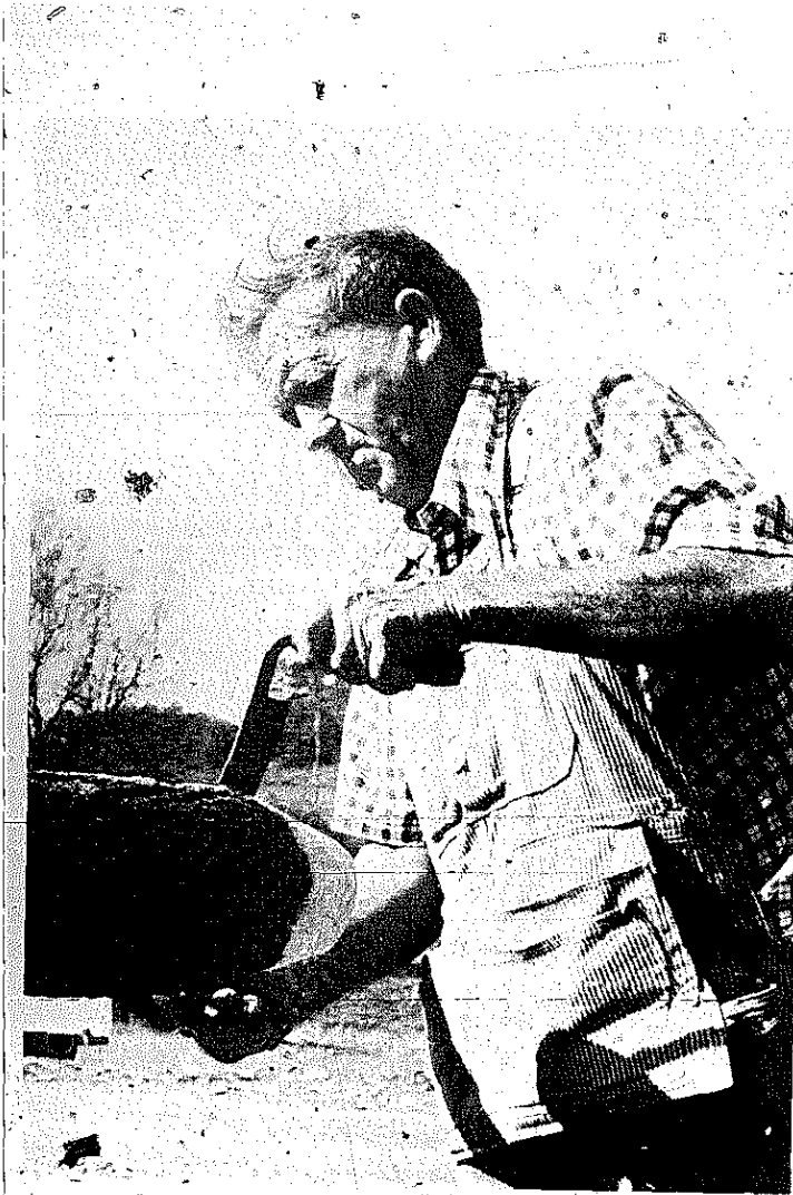
PLATE 313 He then takes another auger and bores a concave hole in the other end of the pipe.
