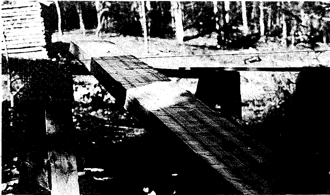
PLATE 410 The finished beam.
