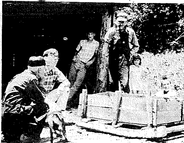
PLATES 193-194 (Variation #4) This sled was made by Harv Reid in Blairsville, Georgia. It has curved sourwood runners and a mortised crosspiece, but the box is nailed to the standards and rests on crosspieces that are nailed to the tops of the runners. In Plate 194, Harv shows where the clevis goes.
