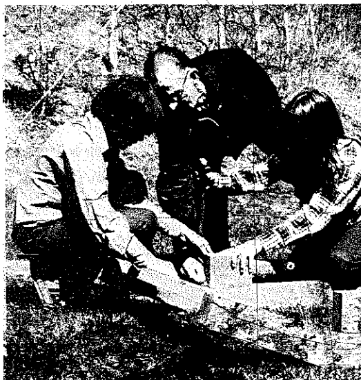
PLATE 165 Cheryl and Dwayne Skenes toenail three chestnut blocks onto each runner. The sills will fit on top of these blocks.
