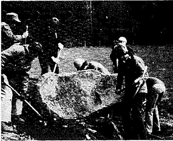
PLATE 251 To turn the rock over we dug the earth out from behind it and rolled it back using poles as levers.
