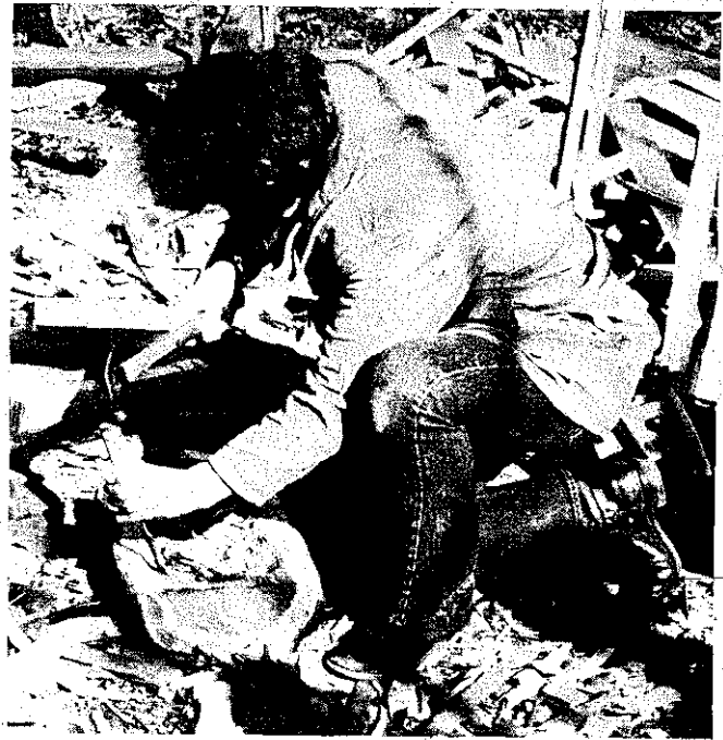
PLATE 108 He also shapes the bowl by using a hammer and chisel as he begins to get closer and closer to the critical points. Here, Roy Dickerson, the author of this chapter, tries his hand at it.
