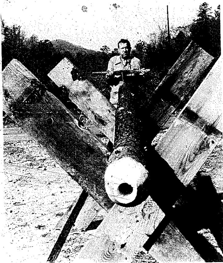
PLATE 311 *To make a twenty-foot section of wooden pipe with a ten-foot auger, Garnett bores into one end as far as the auger will go, and then switches ends. He has to be careful not to let the auger bore out the side of the log as it gets in deeper and deeper. He constantly sights along the shaft to make sure it's going straight.
