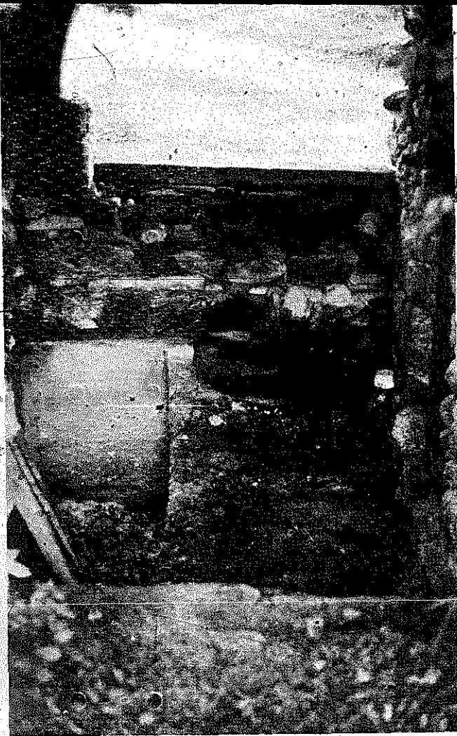
PLATE 335 Point B, view of the steps and water inlets.
