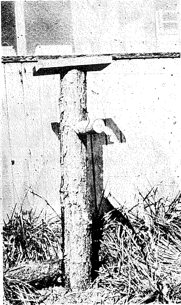
PLATE 315 The finished spigot. The plank on top is nailed firmly in place to prevent the water from shooting out the top through the bored hole instead of the poplar spout in the side.
