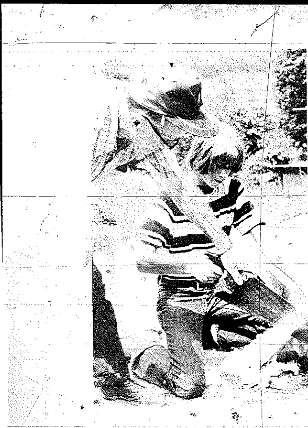
PLATE 175 Then he shows Ken how to cut a series of slots at the spot the pole must bend.
