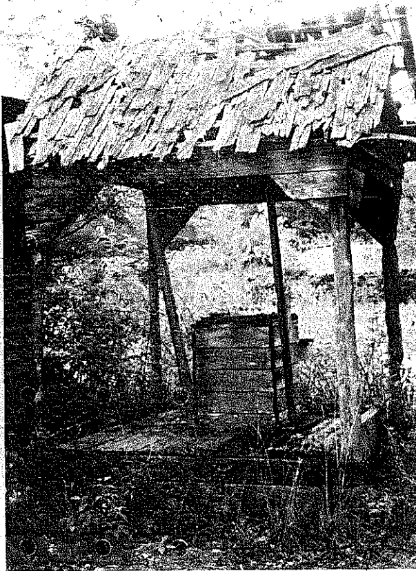
PLATE 347 An abandoned well in the mountains. Note the wooden curb built up over the hole to keep things from the surface from falling into it.
