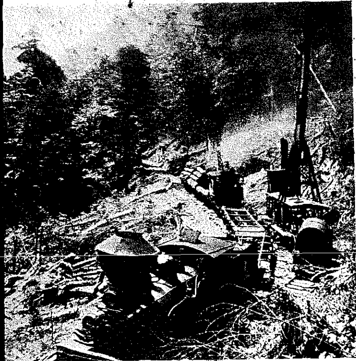
PLATE 277 At the head of the railroad line, an overhead skidder (far right) powered by a steam boiler would be used to drag the logs out of the woods, where they had been cut, to the loading area. There a log loader (or "stiff-necked loader"), visible in this photograph on the tracks beyond the steam engine, would load the logs onto the railroad cars for the trip to the mill. When one car was filled, the loader would pull off the main track onto a short siding so that the engineer of the train could move another empty car into position to be loaded. (Photo courtesy of Champion Paper.)
