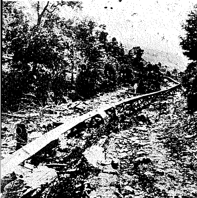
PLATE 271. Acid wood (chestnut) was essential for the production of paper. Companies like Champion International would build miles of flumes up into the mountains in order to get this acid wood out. A flume would begin high in a watershed nearly at the head of the creek. A splash dam at the head of the flume would hold water to be turned into the flume. The chestnut would be cut into five-foot lengths and split up and stacked beside the flume at intervals along its length during dry weather. Then, in wet weather when the stream was running full, water would be turned into the flume at the splash dam and the split wood would be loaded into it and carried to its end. The flume pictured here was on Big East Fork. (Photo courtesy of Champion Paper, a division of Champion International Corp., furnished by C. W. Hardin.)
