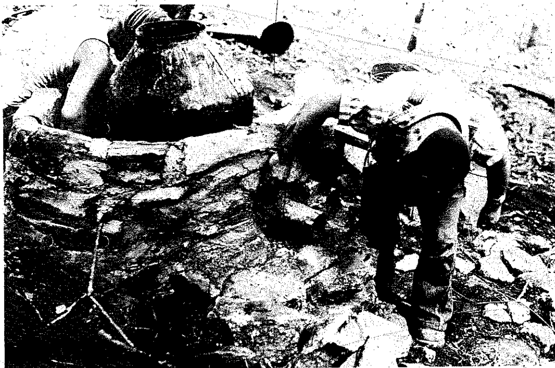
PLATE 437 Then he sealed the hole around the slop arm with red-clay mud while one of the students helped by lining the sloped inside back wall of the furnace with cement and smoothing it up.
