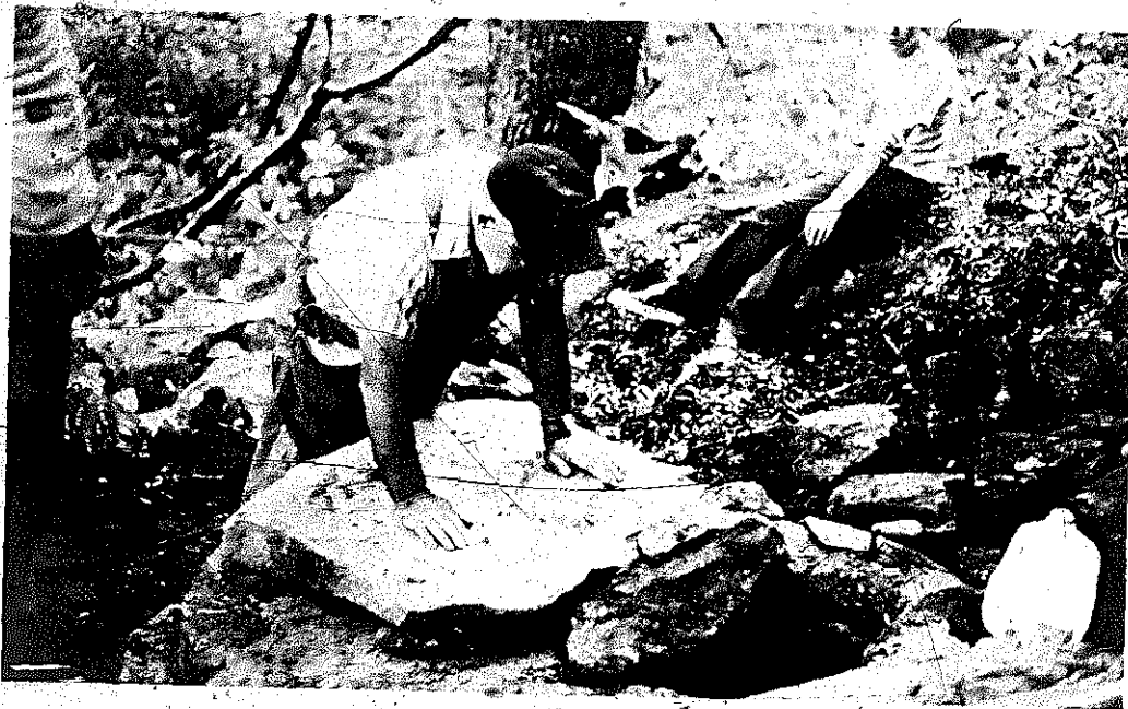
PLATE 429 When the walls of the firebox were high enough (see Plate 431 for measurements), Buck set the large flat rock he had chosen for a bedstone into place so that it spanned the firebox. As it wasn't quite long enough, he set a second, smaller rock into place behind it and cemented the two together to make one flat platform for the still to sit on.
