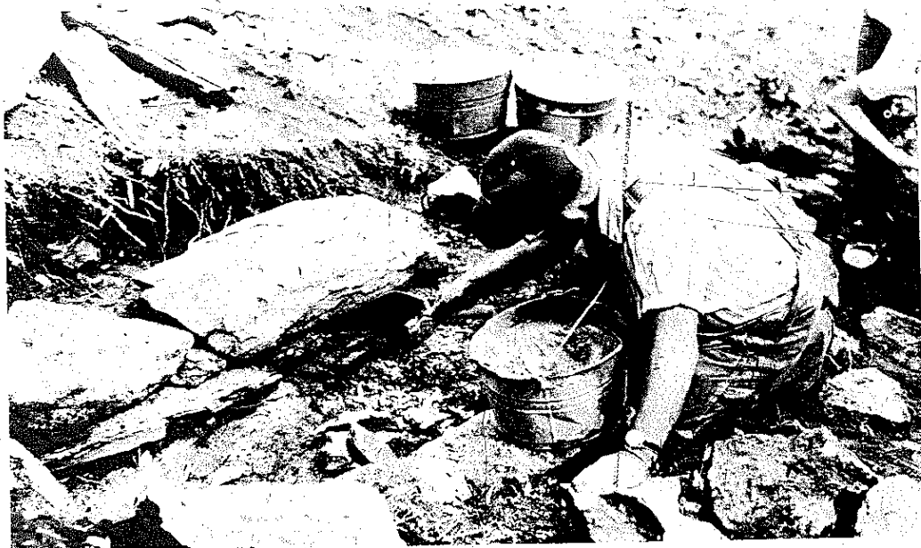
PLATE 428 Next, Buck cemented into place the first two courses of flat rocks thus outlining the firebox walls. Years ago, red clay would have been used instead of cement, and the site for the still would have been partly determined by the availability of clay. In the left foreground, notice that the flat rock at the back of the firebox is set on its edge and sloped backward slightly so that it will deflect the flames upward around the still (see also Plate 431).
