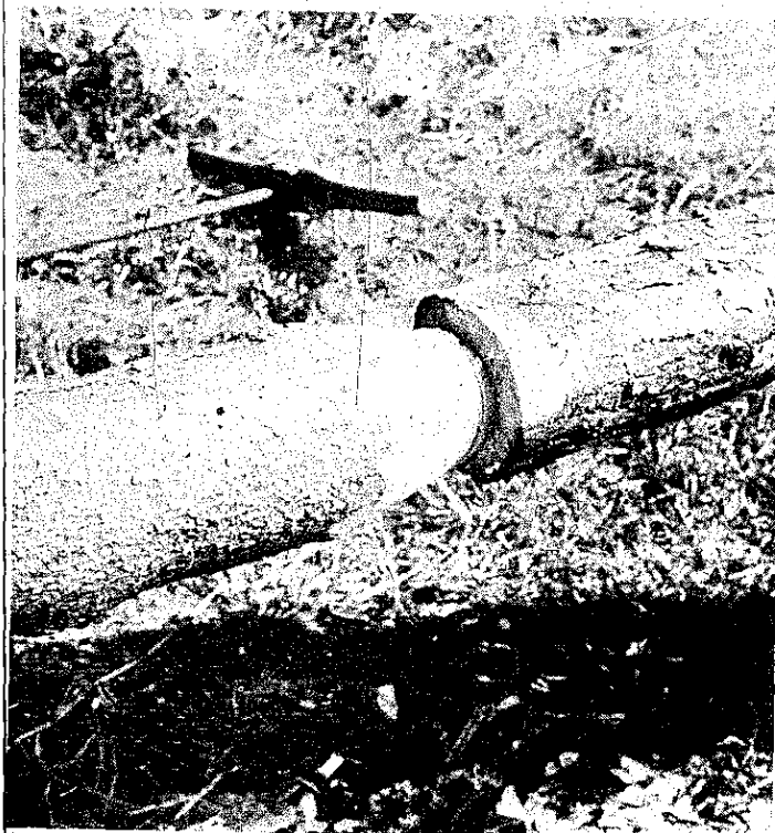
PLATE 314 The tapered end of one pipe fits into the concave end of the next. Just before the pipes are locked together underground, a rag is wrapped around the joint to minimize leaking.
