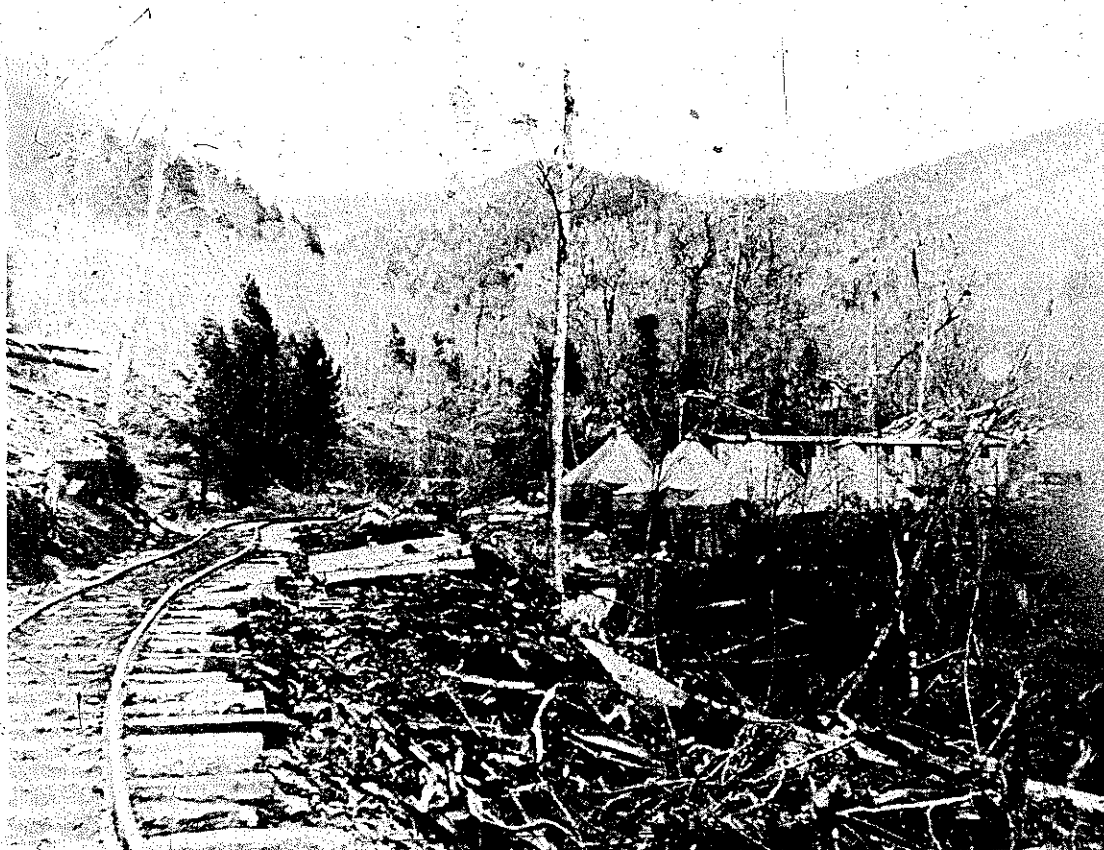
PLATE 287 Another logging camp, this one at the head end of a narrow-gauge railroad line. The dwellings are log sides with canvas roofs. The long, narrow wooden building behind the dwellings is probably the cook shack. An operation like this one might have seventy-five to a hundred men living there at one time. (Photo courtesy of Champion Paper.)
