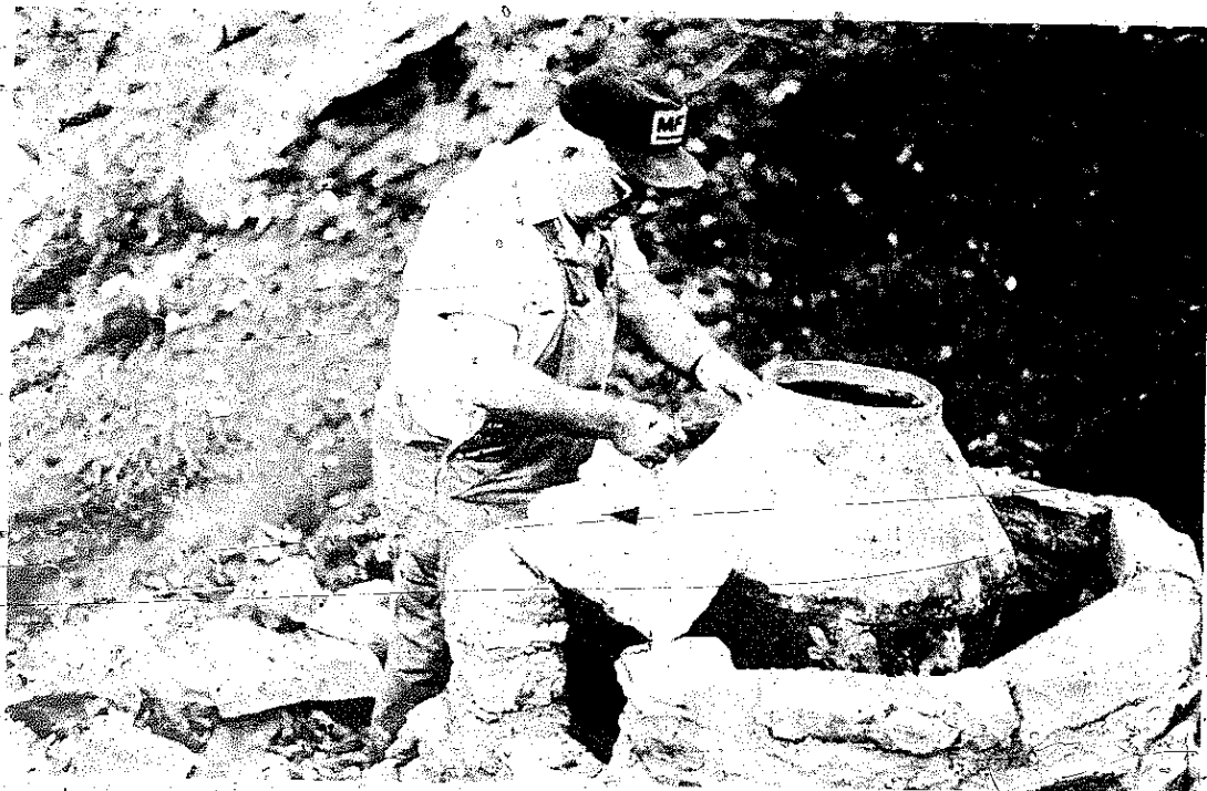
PLATE 438 - Next Buck set flat rocks in place around the cape to form the top of the furnace.
