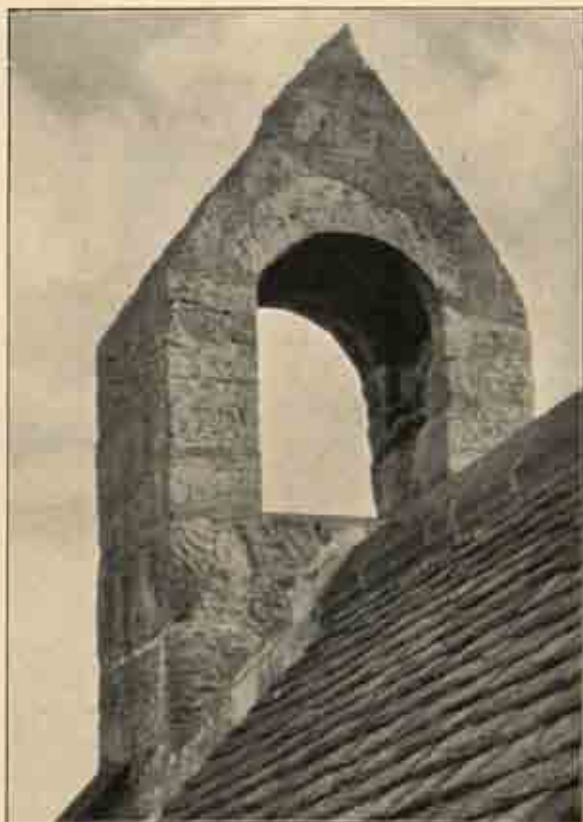
Fig. 10. Thirteenth-century Belfry over Chancel Arch at Abercorn.
