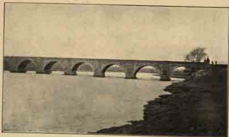
Fig. 5. Bridge of Dee, Aberdeen, 1527.
