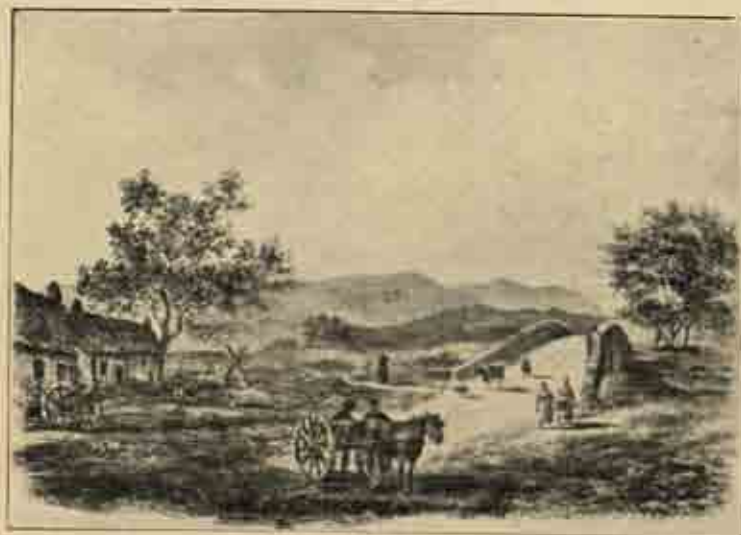
Fig. 15. Millburn Bridge near Moffat.
