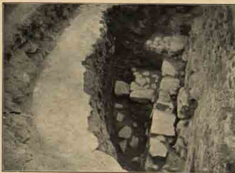
Fig. 11. Pit at Stirling Bridge.
