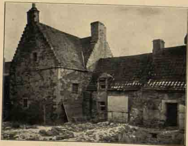
Fig. 2. Back view of Houses at Inverkeithing.
