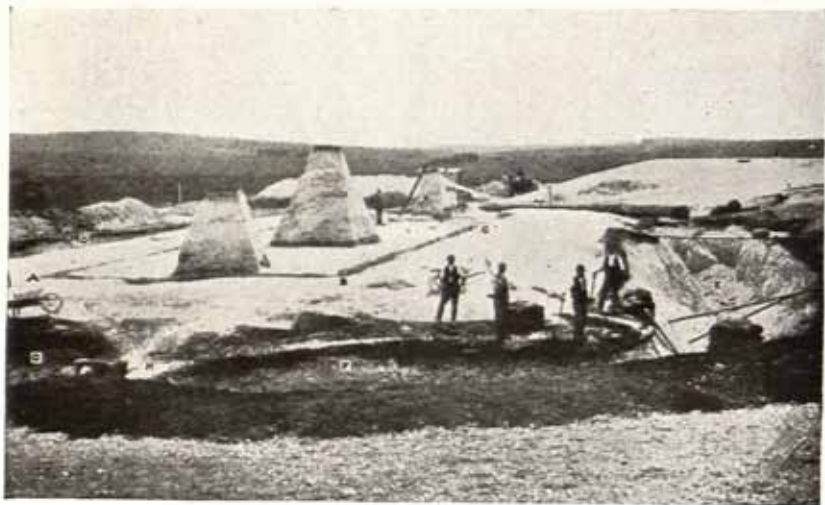
90 WOR BARROW: after excavation
