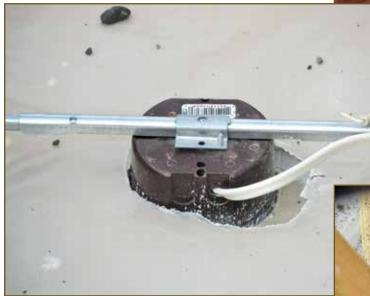
Figure 4 – Vapor retarder bypass at ceiling light electrical box.
