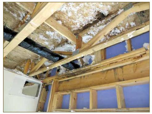
*Figure 6 – Leaky dryer and bathroom vent ducts in truss space.*
