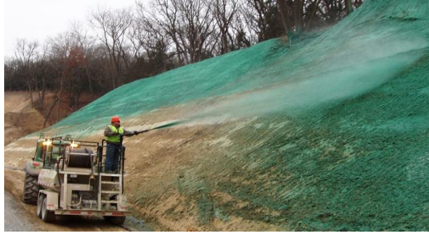
Figure 4: Revegetation techniques with hydroseeding (URL-5)
