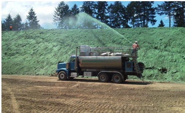
Figure 5: Revegetation techniques with hydroseeding (URL-5)
