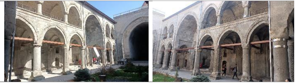
(c) West façade rooms
