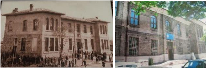
Figure 1-2. Gazipaşa Primary School old period photos, respectively ?-2009, (“Koruma Kurul” archive)
