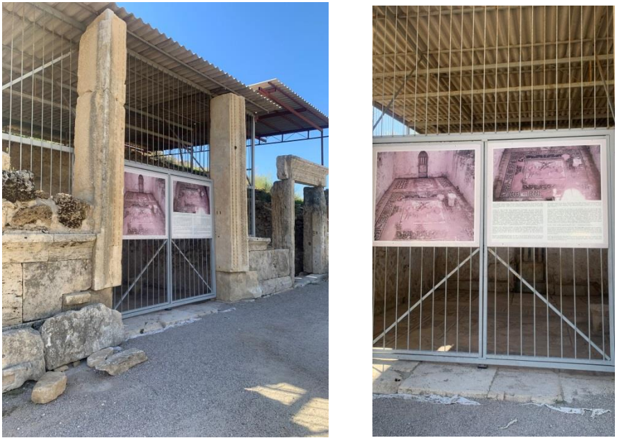
Figure 8, 9. A system designed to protect mosaics from the effects of nature and humans in the Ancient City of Perge (Hattap, 2022)
