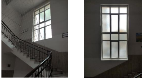
Figure 23-24. North staircase and window
