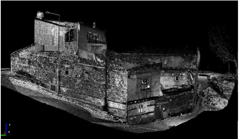
Figure 18: Terrestrial scanning studies (3D Point cloud Data)
