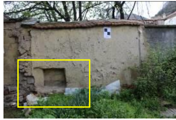
Figure 11. The fireplace in the adobe wall in the south of the garden of the registered house on block 137, plot 32 (From the author's archive, 2018)
