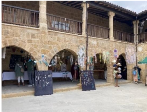
Figure 3. Kumarcılar Han's zoning plan showing the use of spaces after the adaptive reuse and current condition photos (Author, 2023).
