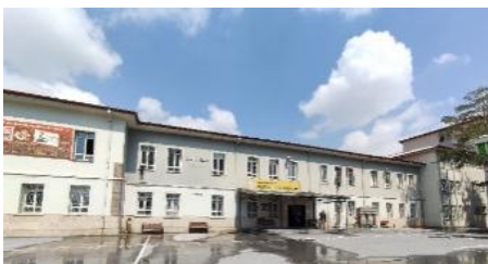
Figure 18. Imamhatip High School South Facade
