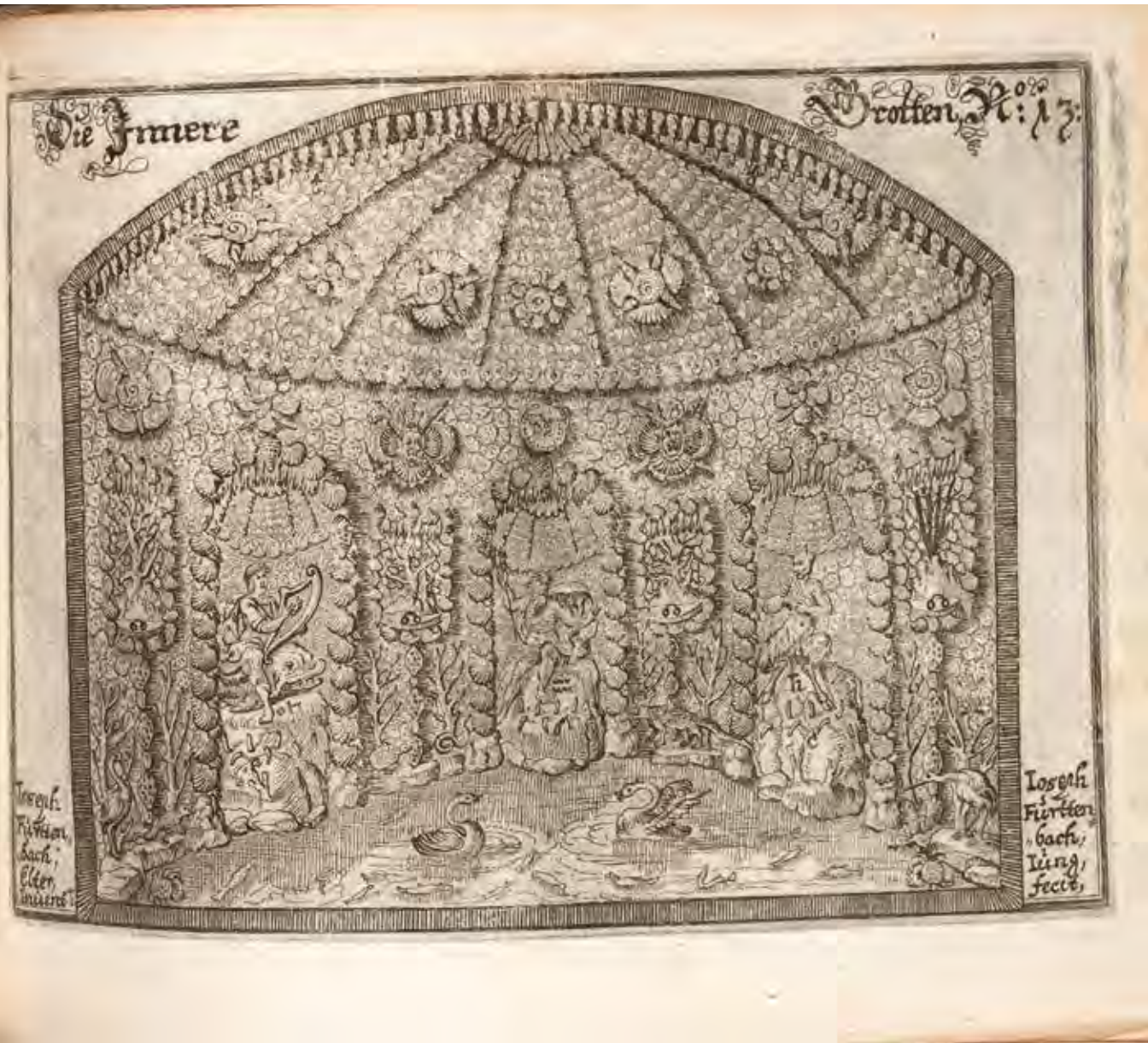
Construction of ornamental grottoes
