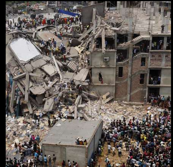
Foto: Jaber Al Nahian/Flickr: Dhaka Savar Building Collapse
