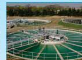
SEWAGE TREATMENT PLANT CHEMICALS
