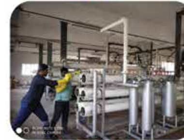
RO Plant Erection
