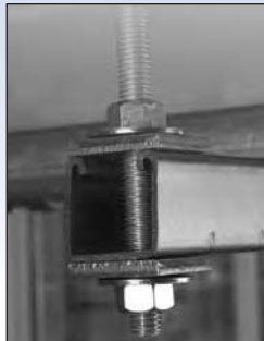
Standard method using nuts and washers.
