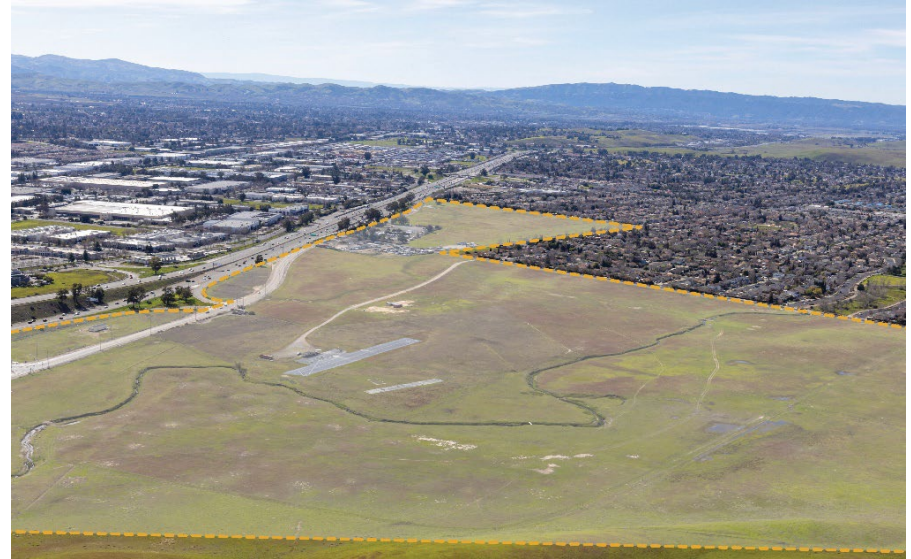
Bird's eye view looking west toward the Laughlin Road Focus Area.
