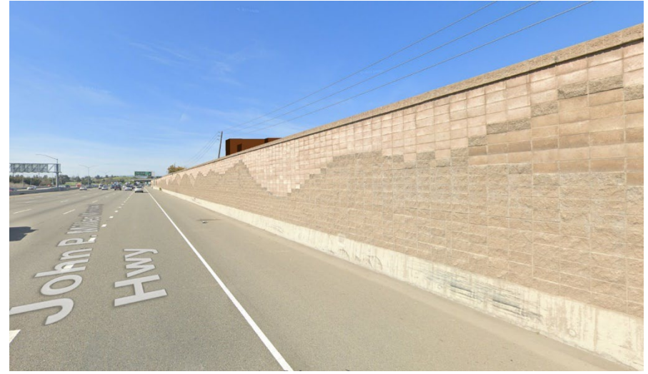
View of the massing envelopes of potential development of the Blended Alternative in the Midtown Focus Area North. The upper stories of high-density residential development would likely be visible to travelers along I-580.
