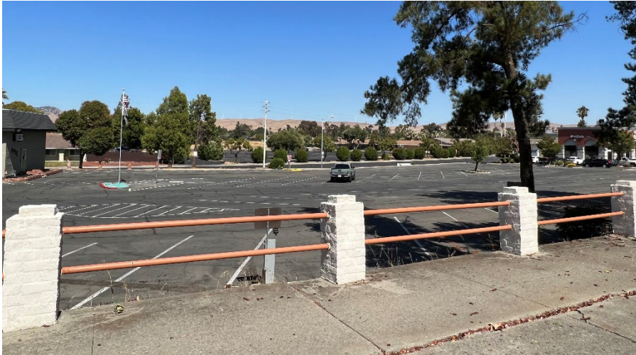
Existing commercial parking on Springtown Blvd lot in the Midtown Focus Area
