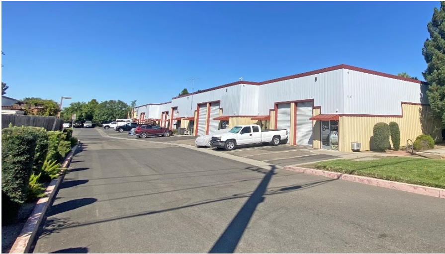
Existing light industrial uses in the Vasco Row Focus Area.
