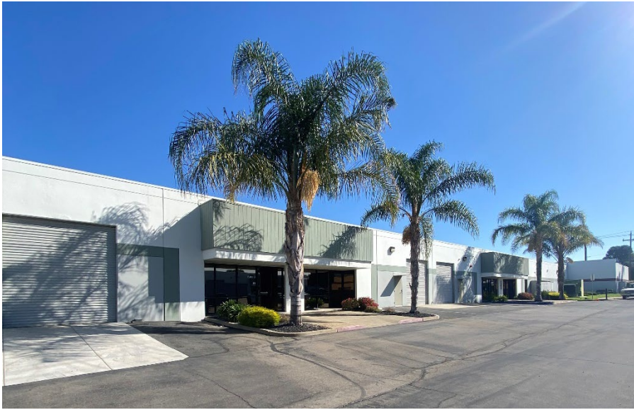
Existing light industrial uses in the Vasco Row Focus Area.
