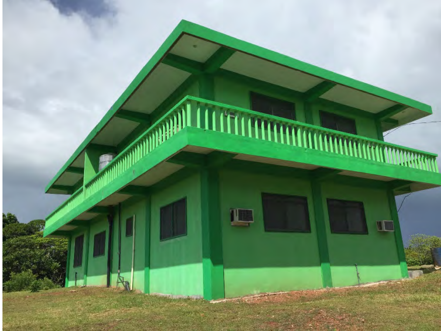
Photo No. 34 – 22 November July 2019 Completed construction of the new house on the subject property at the Ngaraard Tx Site. Looking north.
