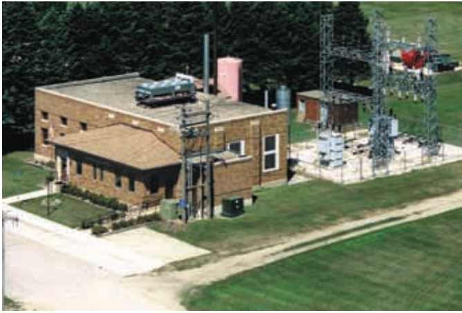
The Cummins Power Generation standby system installed by the city of Graettinger provides power for residents if grid power is lost.
