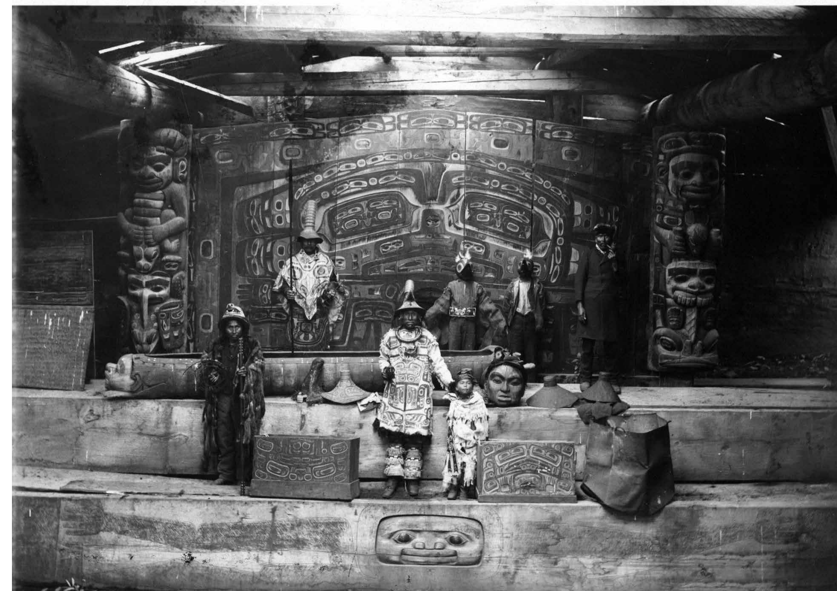
Interior of Klukwan Whale House, circa 1895. Tlingit clan houses were rectangular in shape with a post and beam construction. The more important houses were partly subterranean with one or two step-like platforms descending to a central square enclosure from 4-6 ft below the surface of the ground. This photo of the Klukwan Whale House of the Gaanaxteidi (Raven) Clan shows many Clan and House treasures.
