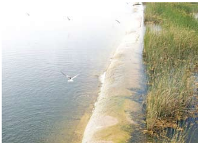
Fig. 3. A weir with convex crest/top. Water flows in the form of thin film across the weir from the marshy wetland of Bhaskarpura (on right hand side) to a pond-like waterbody (on left hand side).
