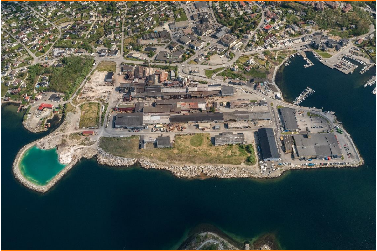
Production Facility, Jørpeland Norway
