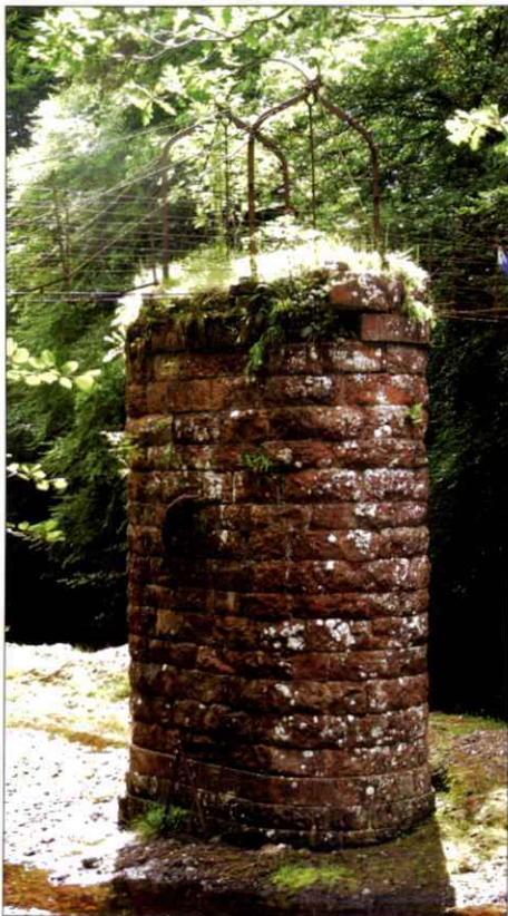
right, Louns Bridge pier and remains of bridge
