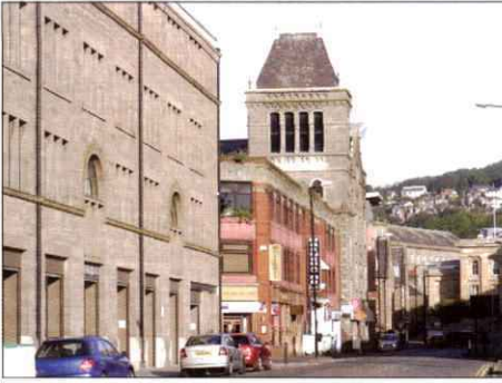
D3 Dundee House, left, and D2 Lindsay Street Mill
