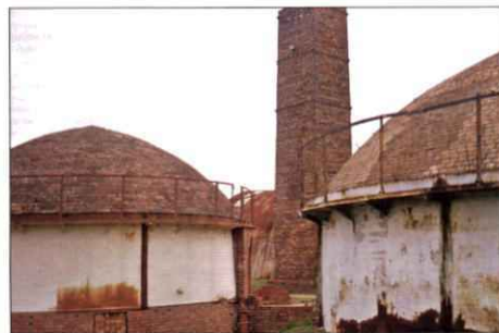
CG4: Errol brickworks, two beehive kilns and a square chimney
