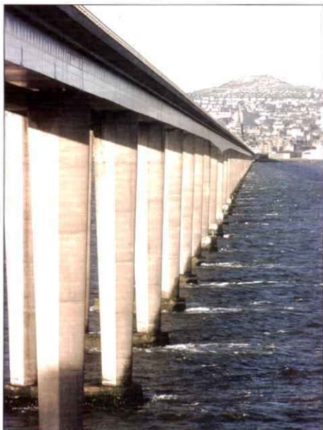
DD3: Tay Road Bridge, looking towards Dundee
