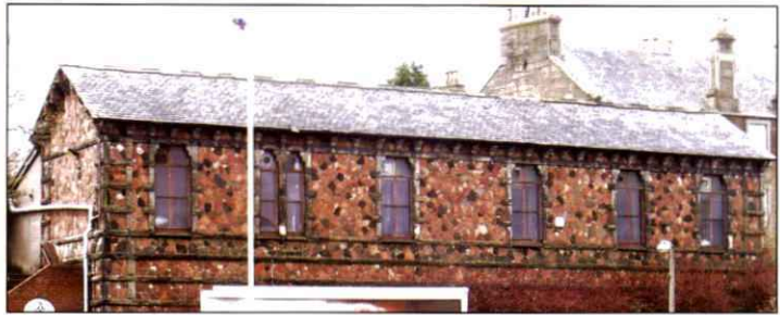
DW3: Lochee station and (left) corner detail of stonework
