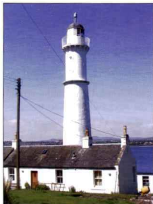
F24: High and Low Tayport lighthouses by Robert Stevenson, one taller than the other to line up with the navigation channel. Built by Dundee's own Trinity House in 1823. The taller (left) 24m/77ft high tower is whitewashed as a day mark. The lower (centre) 12m/39ft tower has not been lit since 1848 when it was supplanted by F25 (right), built on timber piles by James Leslie. Associated keeper's cottages which with the lights are privately owned.
