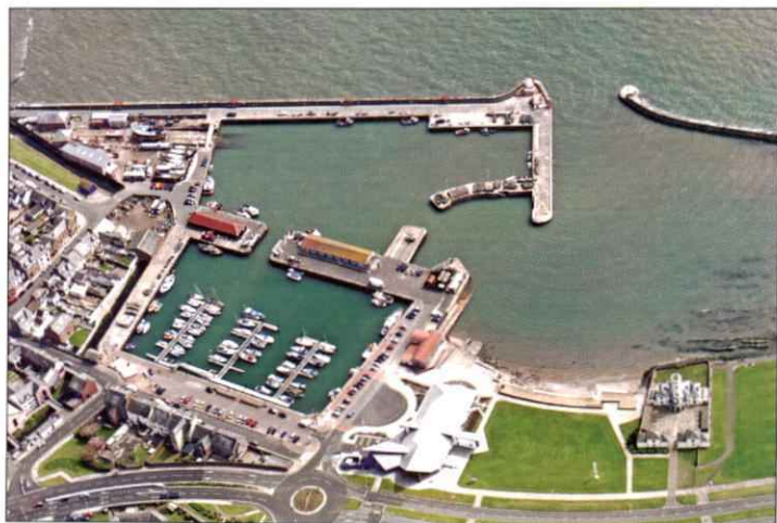
AR6: Oblique aerial view of Arbroath harbour and AR7, signal tower, bottom right, patent slip and MacKay's yard top left, 2008
