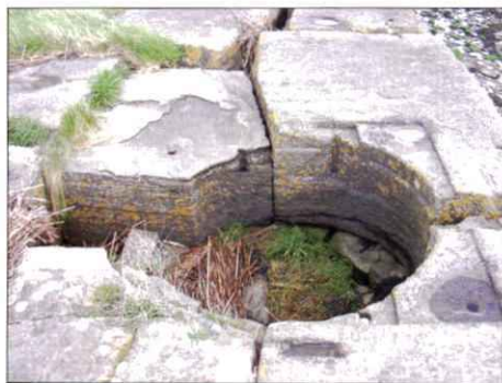
left, CG1: Bullionfield paper mill above, CG2: Kingoodie Quarry, socket for wooden crane in quayside, formed in Kingoodie stone
