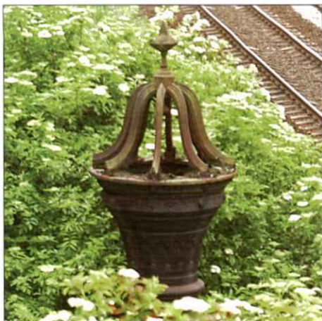
DD10: Sewer Ventilator, Dundee
