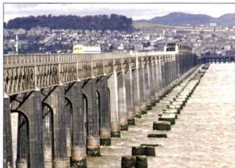
20 DW15: Tay railway bridge with the remaining foundations of the first bridge to the right.
