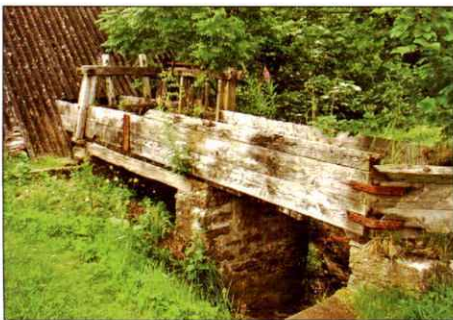
right, AN12: Water wheel at Glamis Mill below, AN12: the Mill launder
