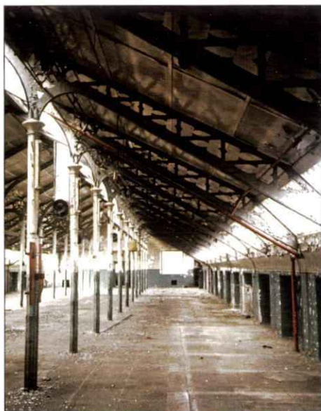
DE9: Eagle Mill. This pattern of Gothic-traceried cast iron roof, made in Baxter's Foundry is present in all four spinning mills in Dens Works and at Verdant Works, DW18.
