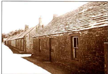
AN13: Douglastown millworkers cottages, the nearest having a local 'grey slate' flagstone roof
