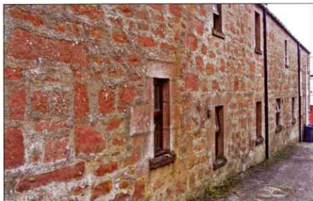
AN5: Blocked window (on left) in former loom shop
