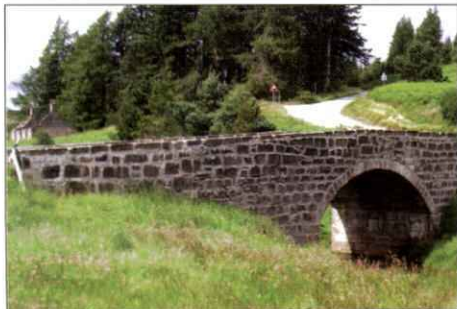
above, M4: Spital Bridge right, M5: Bridge of Dye
