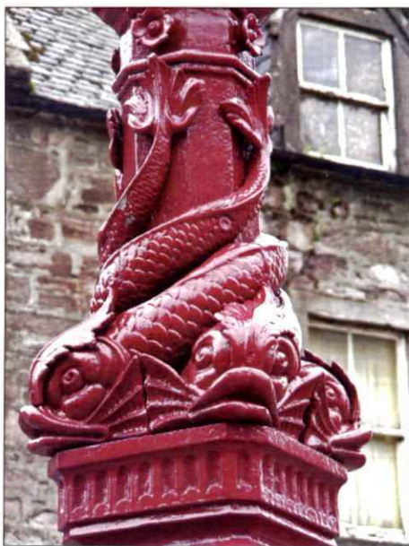
AN28: An ornate cast iron lamp standard in Brechin, by George Smith of Sun Foundry, Glasgow
