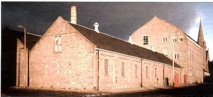
DE14: Arbroath Road, Taybank Works weaving shed
