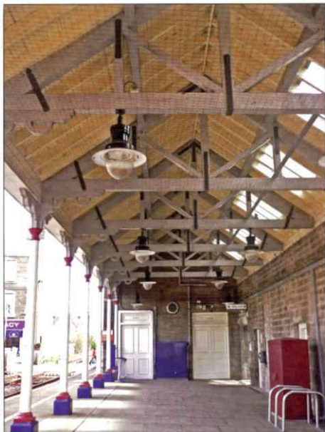
DG19: Broughty Ferry Station
