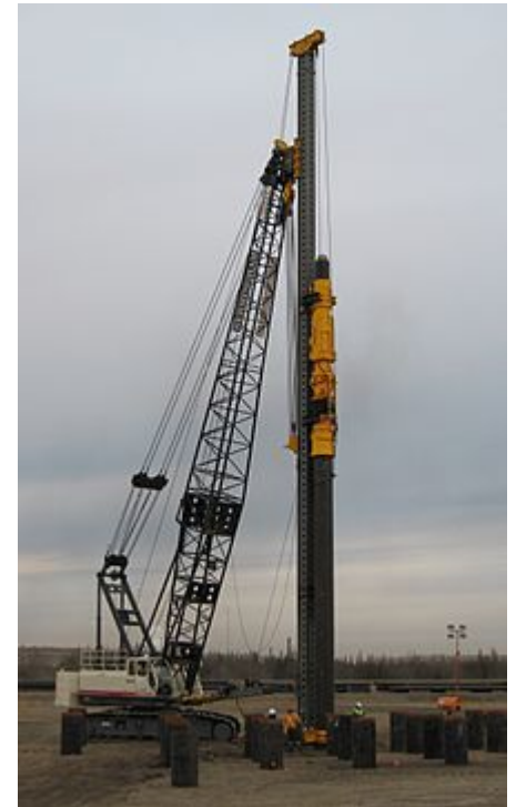
Pile driver: analogy to the nailer (larger scale)
