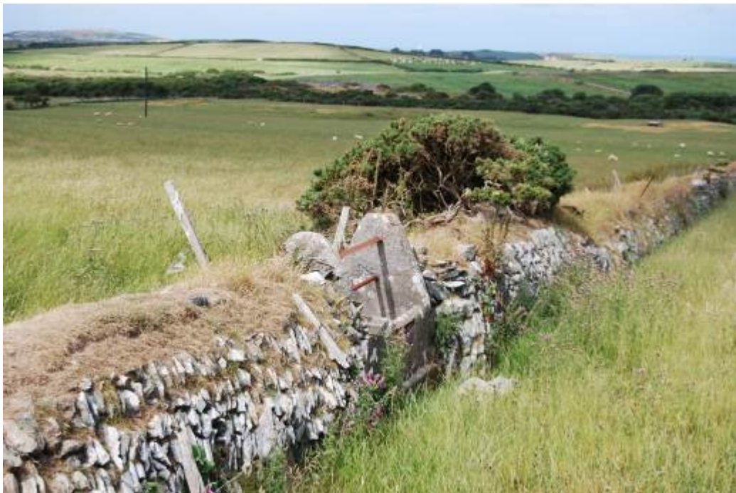
Photograph 9: Example of a traditional field boundary. The wall is in good condition with some turf remaining. Scrub (hedge) vegetation is sparse.
