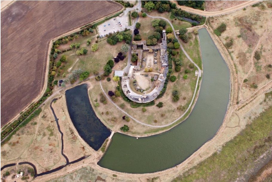
Plate 10 - Coalhouse Fort (Site 48) (EX16/03/056 © Essex County Council)
