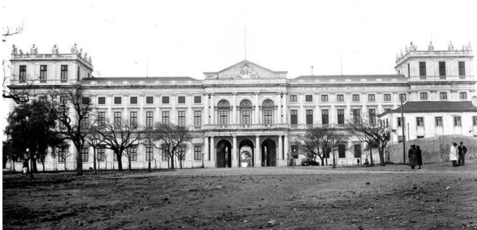
Fig.1 The Palácio Nacional da Ajuda at the beginning of the 20 th century.
