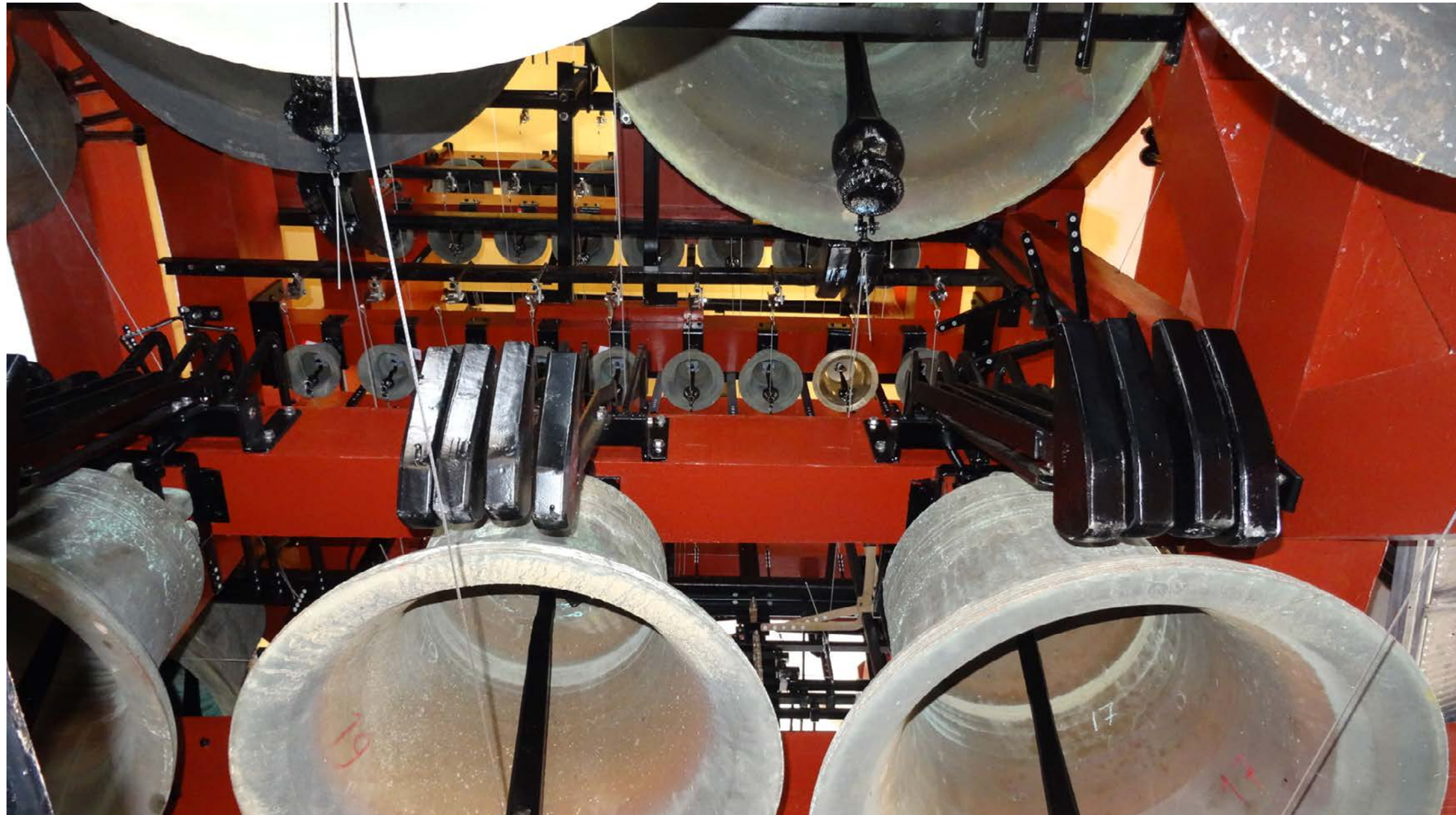
FIG. 6. Bells of the South Tower © Filipe Ferreira — AOF
