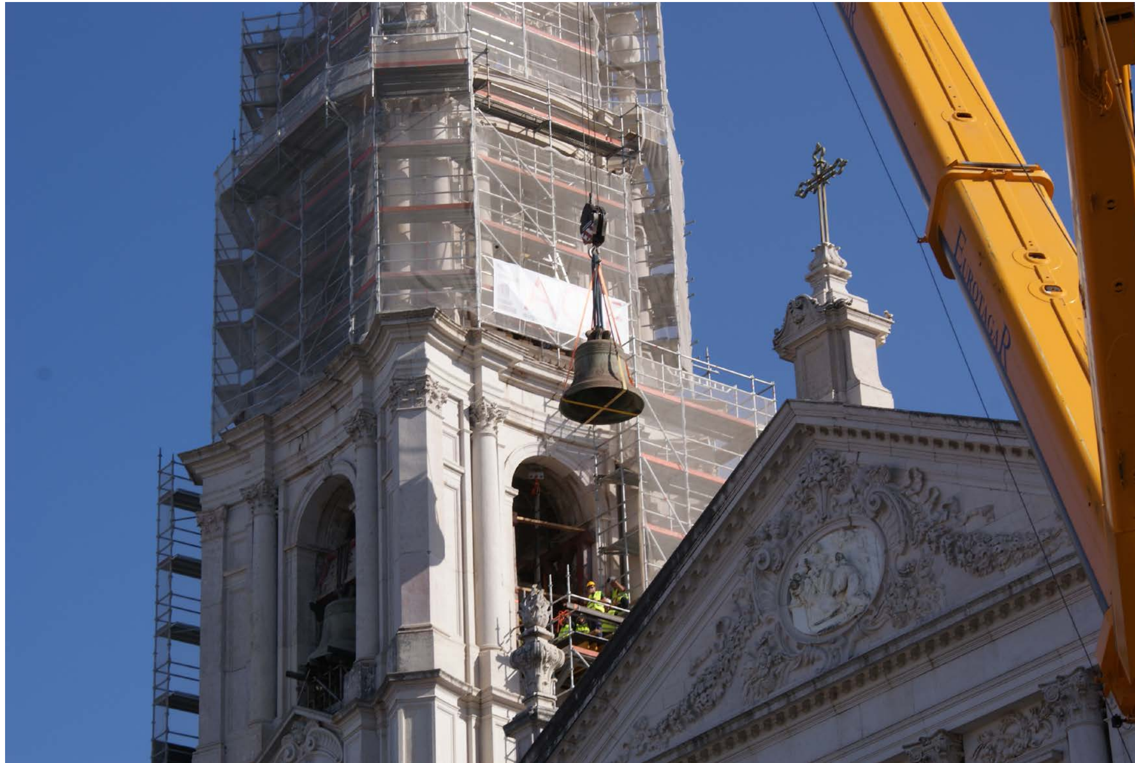
FIG. 8. Bells “that flew through the air...”. 2019 restoration © Filipe Ferreira — AOF
