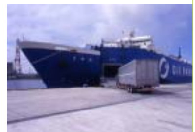
Berth at Tomakomai Port
