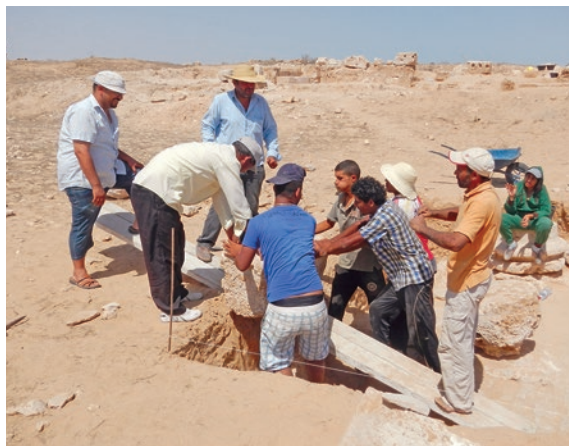
The removal of a large architectural element from the excavation unit in the forum at Zita (Tunisia) as discussed by Ali Drine.
