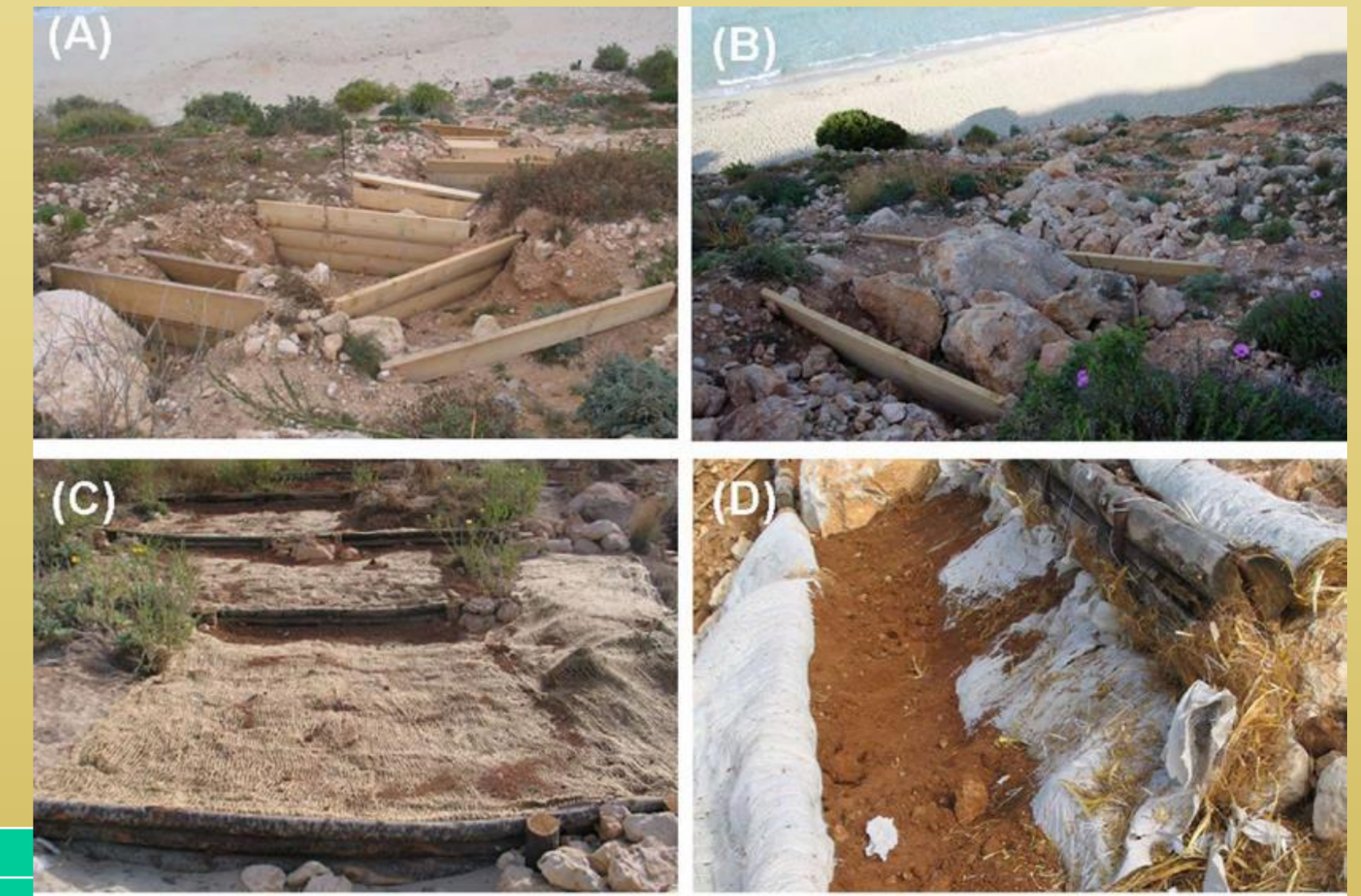
Figure 1 - Some details of the different bioengineering techniques applied at Isola di Lampedusa: woody fences (A), woody fences filled with stones (B), felt mats (C), vegetative pockets made of biomat (D).
