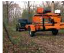
Drive mill to worksite.
