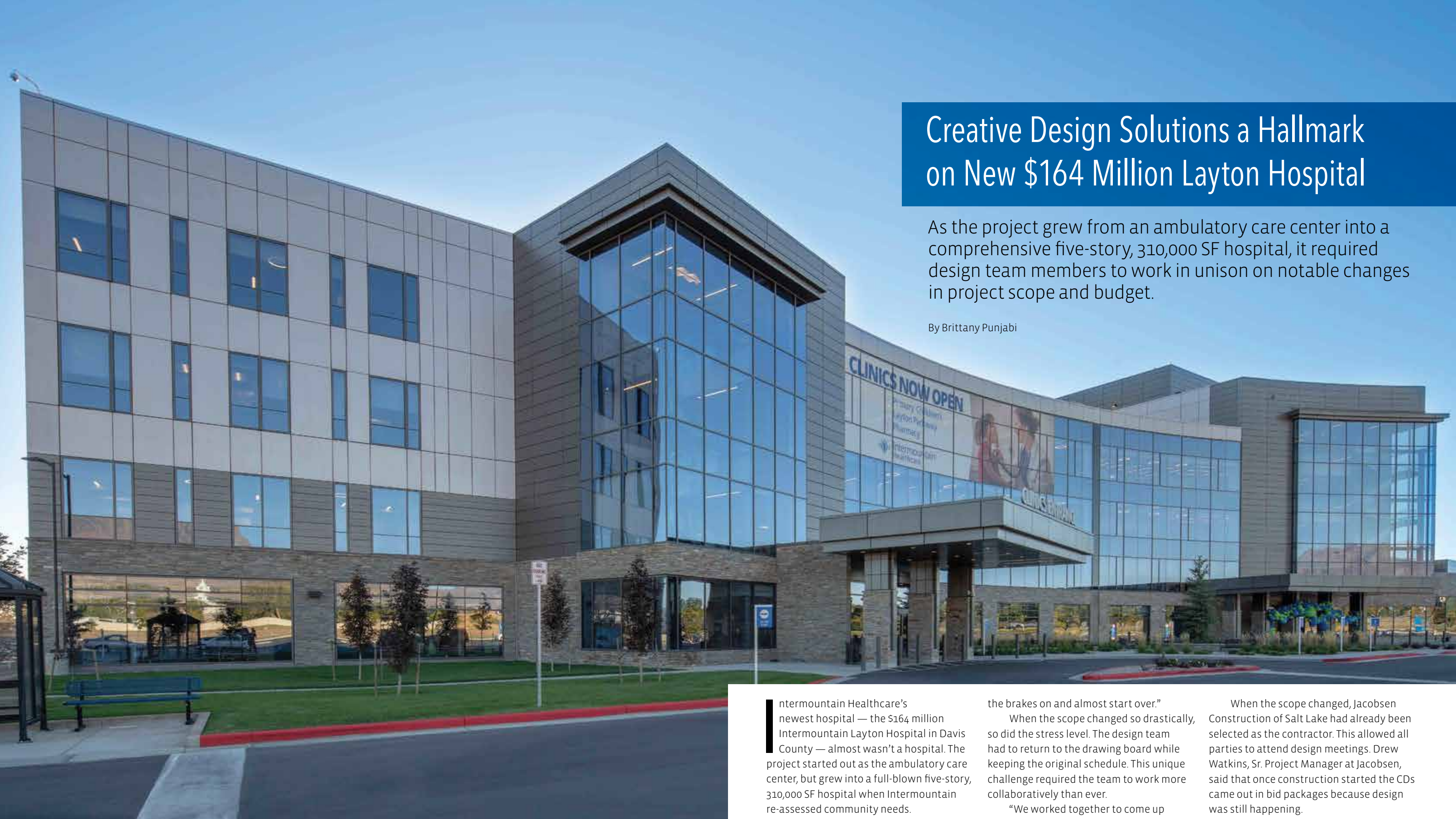
The state-of-the-art, $164 million, 310,000 sq. ft., five-story Intermountain Layton Hospital, that almost wasn't a hospital. (Photos by Jared Kenitzer, Spectrum Engineers)
