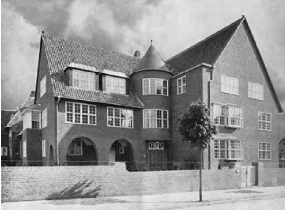
The headquarters building of the Army's intelligence section in Berlin at Ehrenbergstrasse 26/28
