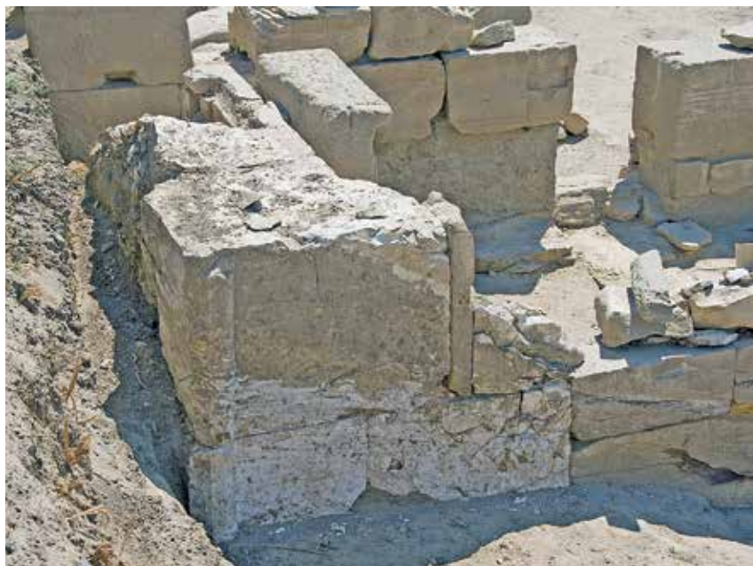
Figure 6.10. View of northwest corner of Chapel D at Mut temple showing the limestone blocks reused in the Ptolemaic era (photo by Betsy M. Bryan)
