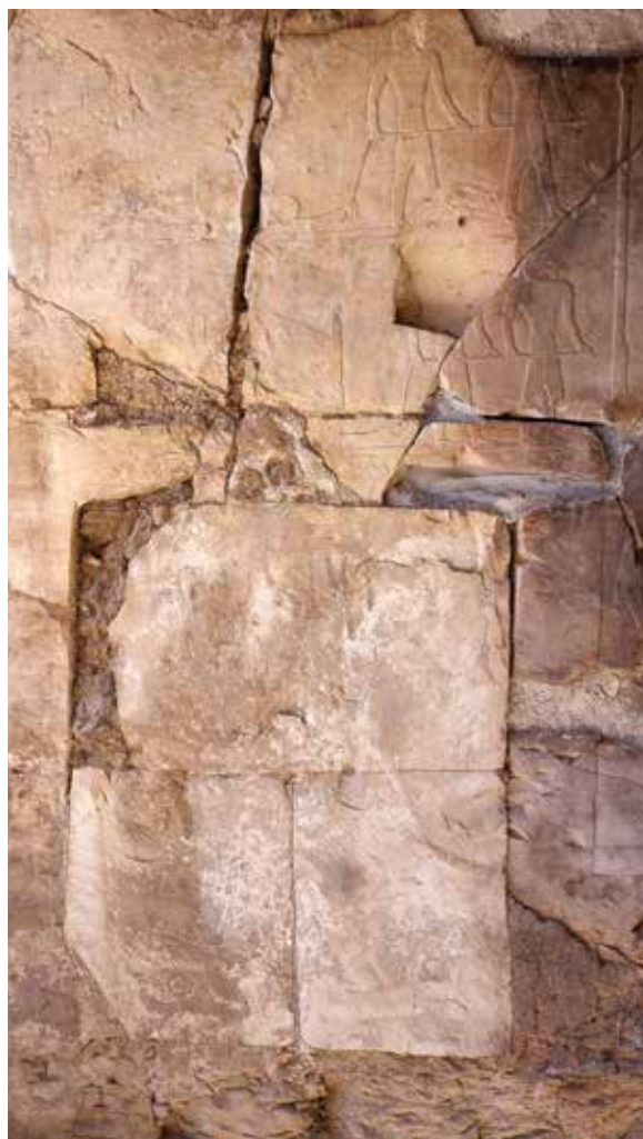
Figure 4.23. Masonry limestone blocks embedded in the left-hand/southern wall near the entrance.
