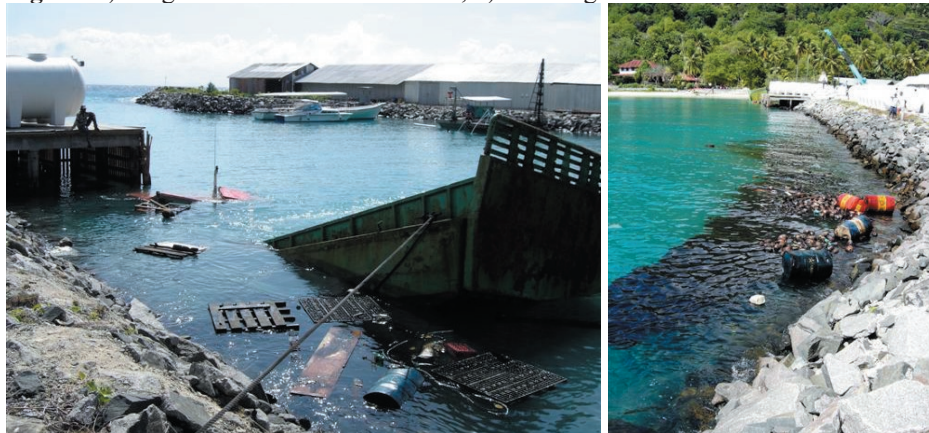
Fig. 18. a) Barge sunk in La Passe harbour, b) oil along the harbour walls
