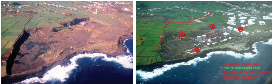
FIGURE 13. A, The quarry at Cabo da Praia on Terceira in 1995 and B, in 2006. (Photo's courtesy of J.A. Paulus Bruno).
