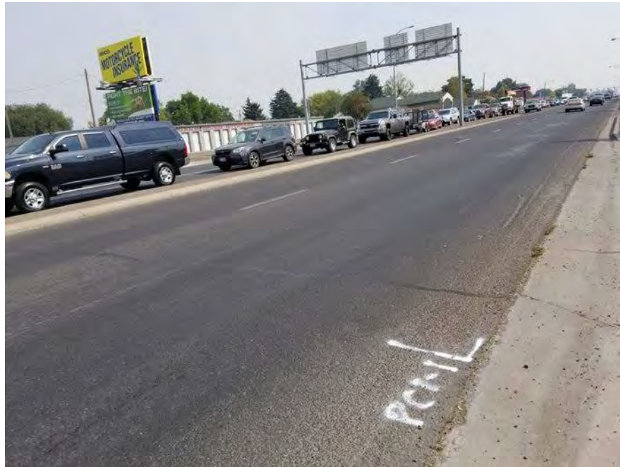
Photo 1: US-30, MP 218.65. Westbound Lane.
