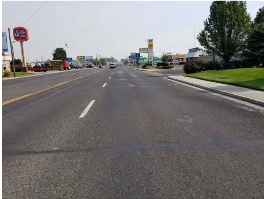
Photo 5: US-30, MP 219.25. Westbound Lane.
