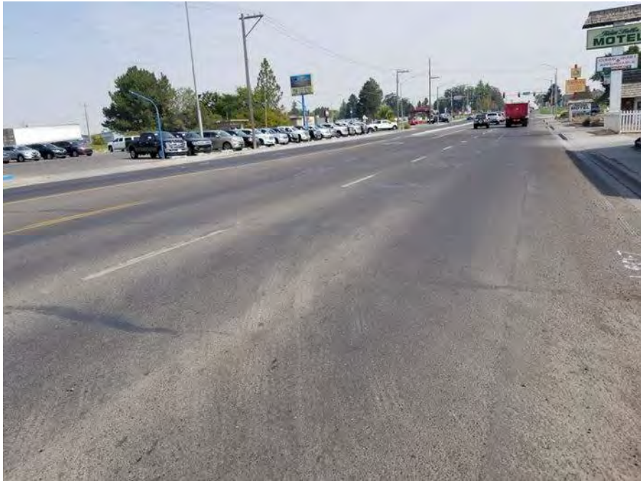
Photo 7: US-30, MP 219.55. Westbound Lane.
