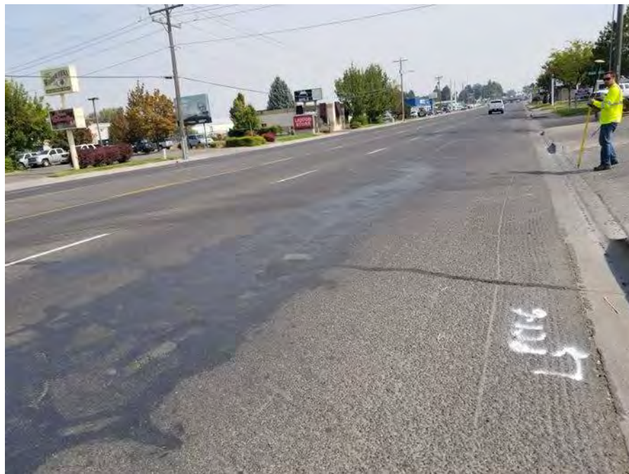
Photo 6: US-30, MP 219.40. Westbound Lane
