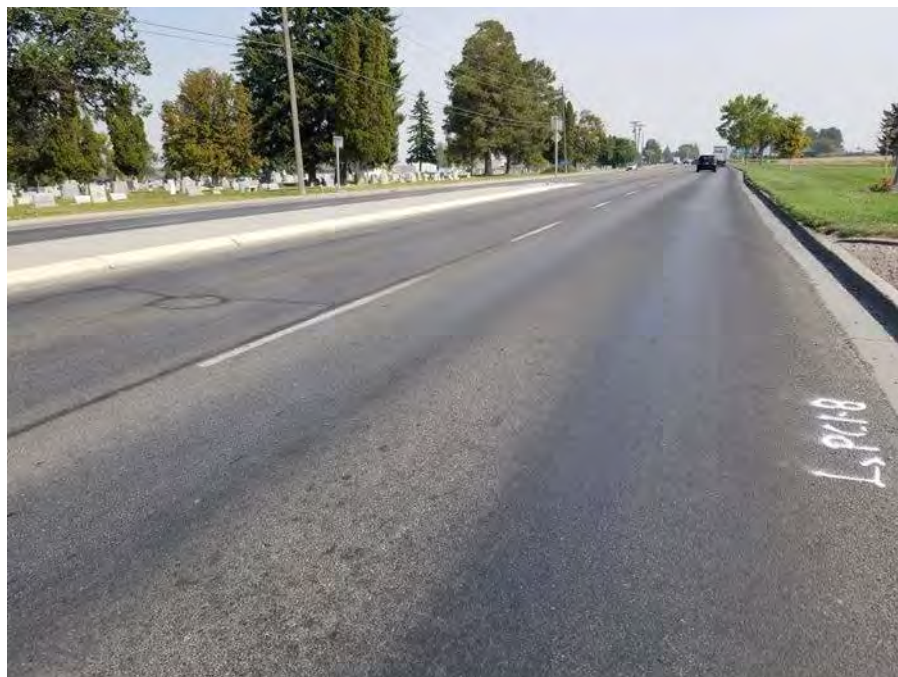
Photo 8: US-30, MP 219.75. Westbound Lane
