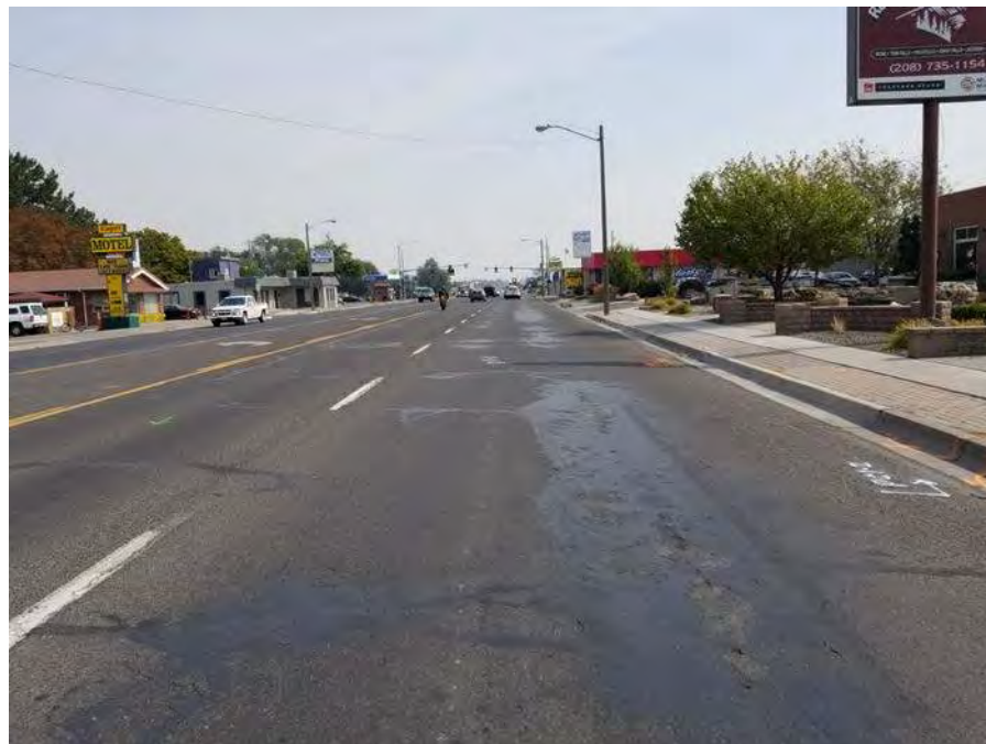
Photo 2: US-30, MP 218.80. Westbound Lane
