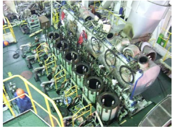
Main engine with all pistons removed
