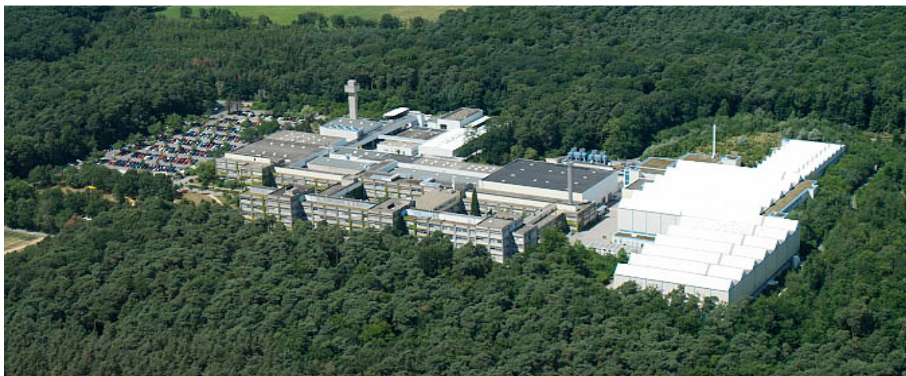
Fig. 4.108.1: GSI Helmholtz Centre for Heavy Ion Research in Darmstadt, Germany. (Used with permission from: GSI Helmholtzzentrum für Schwerionenforschung) [654].
