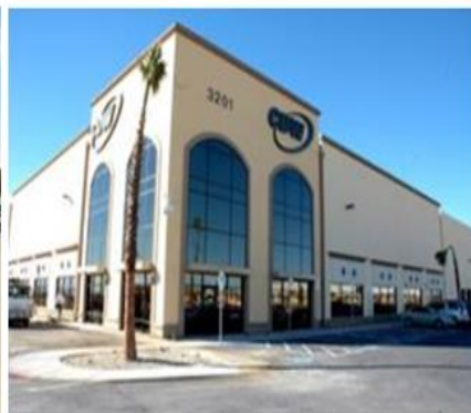
513,000-square-foot distribution center in NV
