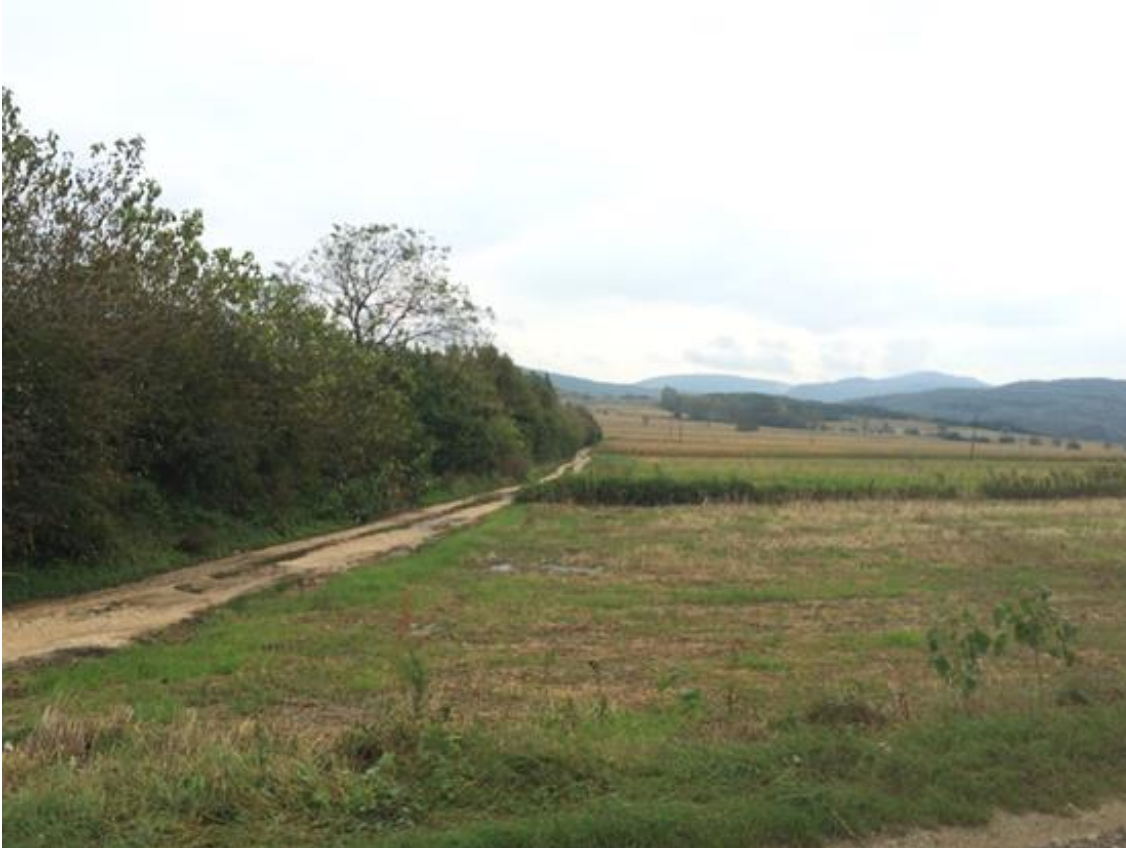
Figure 6: Example of an existing access track which will be upgraded for the Project
