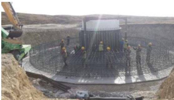
Figure 7: Example of anchor cage being installed
