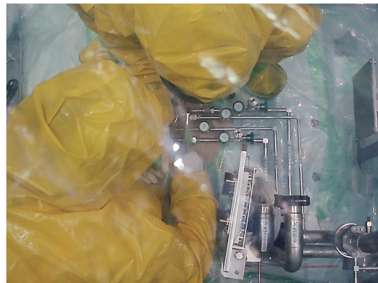
Figure 2. The utility pipes of the PBW were removed manually. The workers were equipped with airline masks and anoraks, and worked in the greenhouse.
