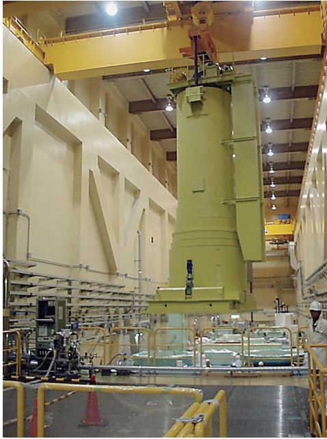
Figure 3. PBW is stored in the shielding cask and moved to the hot cell with a 130-t crane.
