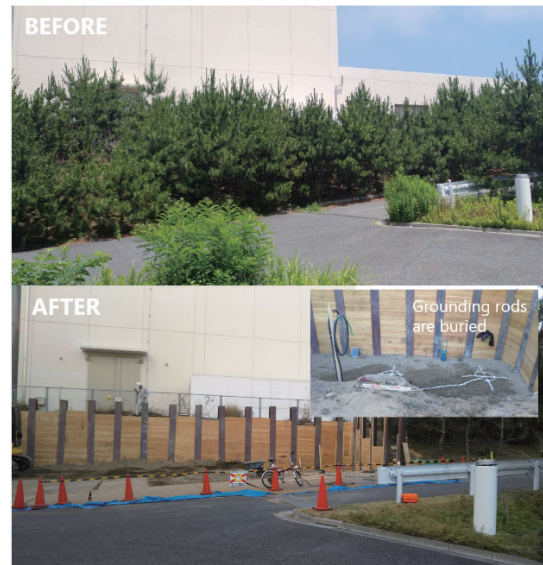
Figure 4. Recent progress of the construction of the electric power sub-station.
