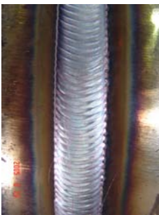
Finished weld / Capping pass
