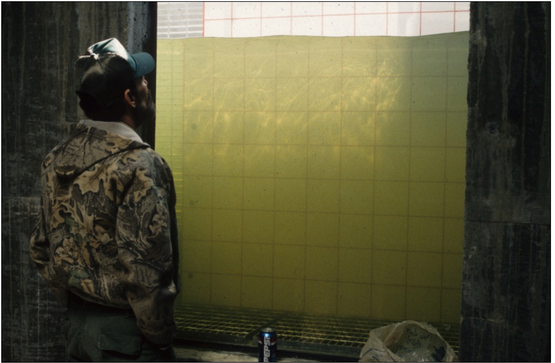
The fish ladder at Boshers Dam has a viewing window to monitor migration of anadromous fish.
