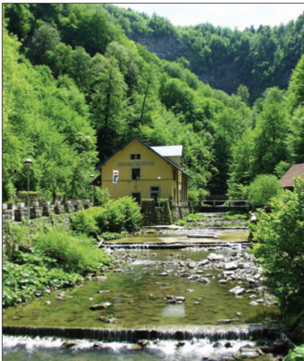
■ The small Munjara hydroelectric power station, built in 1921, is a kind of monument of technical culture.
