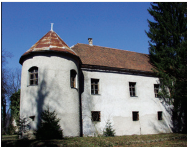
■ The old castle in Severin na Kupi.
