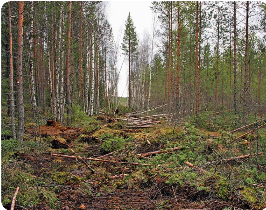
Ditches are infilled with ditch spoil and peat from between the ditches. PHOTO: JOUNI PENTTINEN
