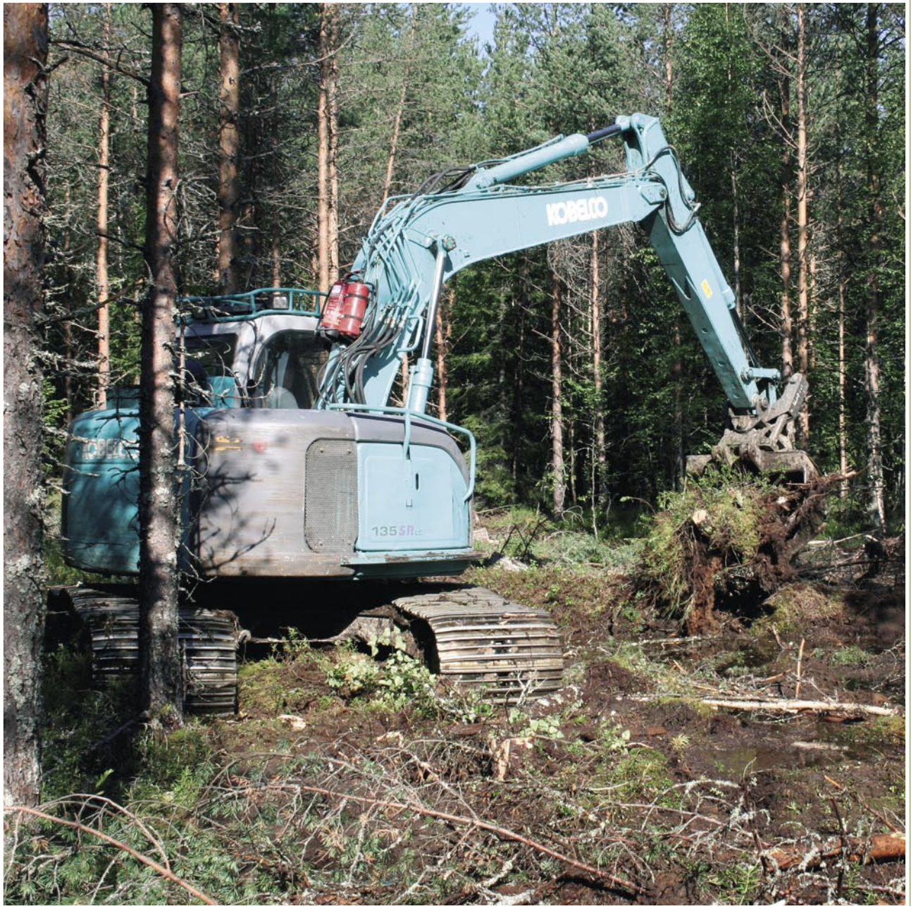
An excavator doing restoration work in a forest-covered mire. Photo: Maarit Similä
