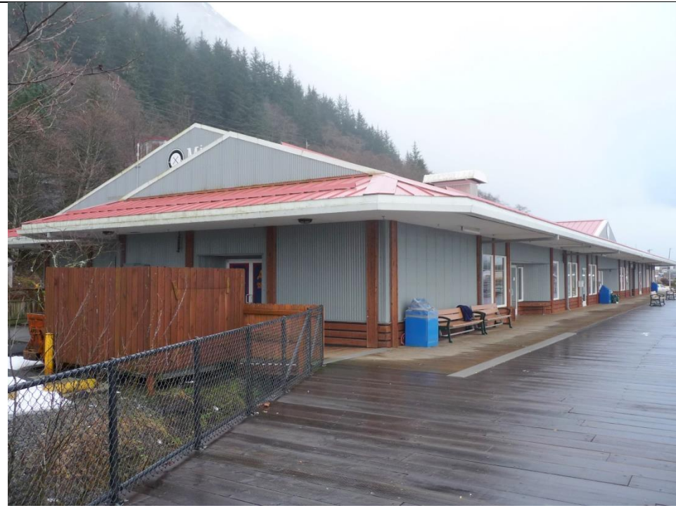
Dock Side – Looking South
