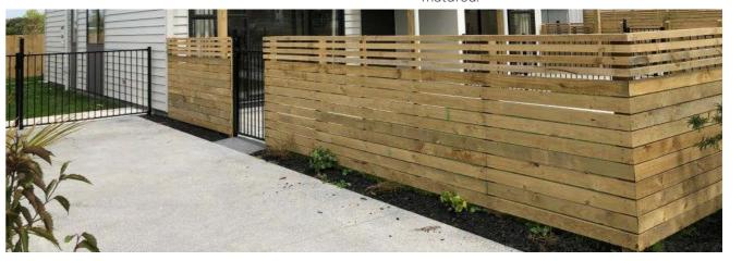
Horizontal slatted timber fence with a 300mm permeable top.
