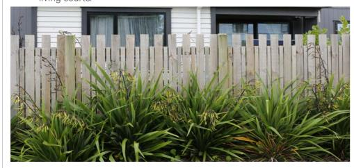
1200mm timber batten fence along a common accessway.
