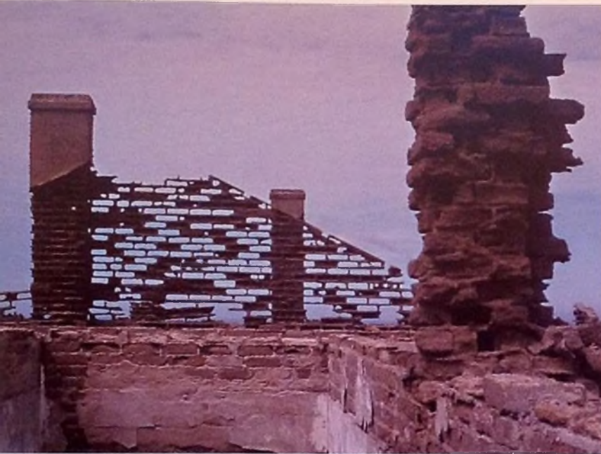
The remains of a wall of one of the houses at Elizabethbucht in the diamond area south of Lüderitz, in 1976. The effect of the frequent sandstorms can clearly be seen, with the bricks having been completely removed, leaving only a latticework of mortar. Photograph: Rodney Moffett
