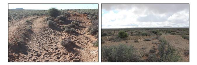
Left: A poorly maintained road, with severe erosion caused by excessive runoff resulting in it becoming unusable. A new road has then been made alongside it. Right: A well maintained road. The well-constructed berm diverting water is visible, and the centre line is mostly vegetated. (*Images supplied by Bonnie Schumann*)
